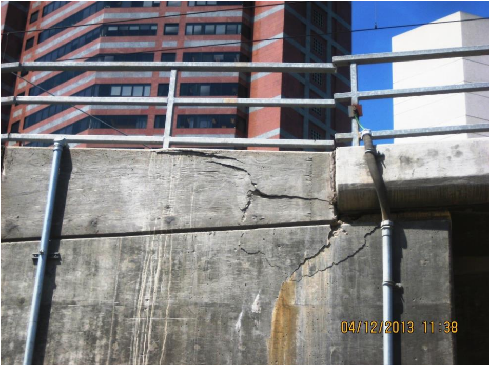
Before Repair (April 12, 2013):
