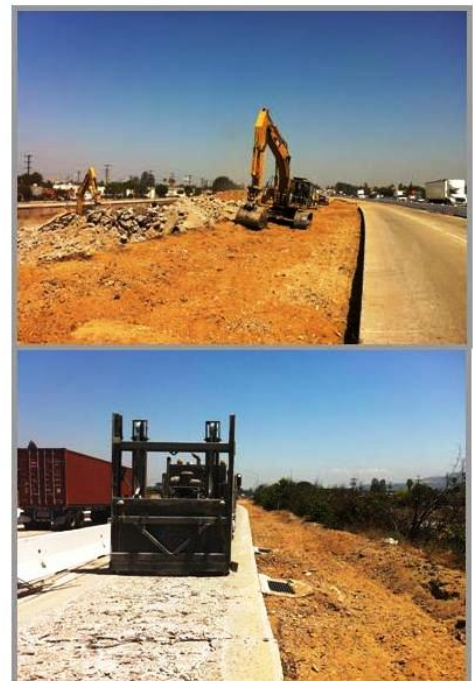
Removal of concrete on southbound I-5.
