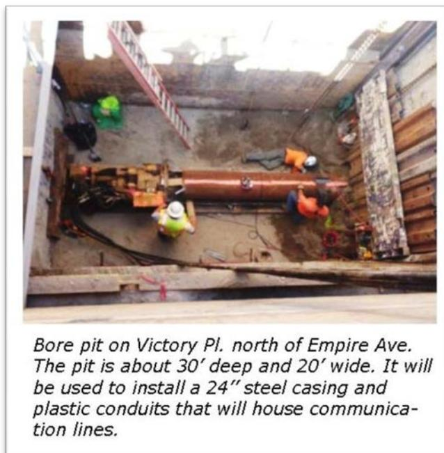
*Bore pit on Victory Pl. north of Empire Ave. The pit is about 30' deep and 20' wide. It will be used to install a 24" steel casing and plastic conduits that will house communication lines.*
