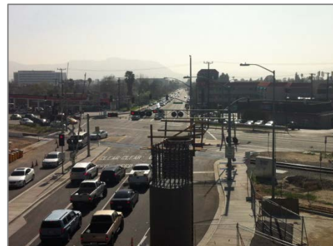
New columns on southbound side of Buena Vista Street.
