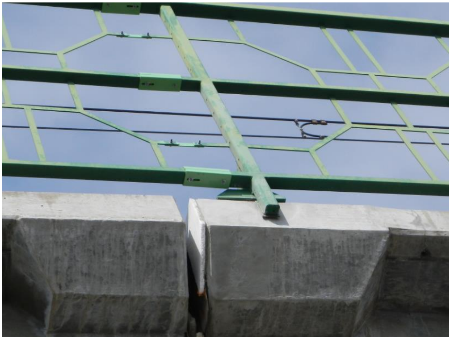
After Repair. (October 17, 2014):
