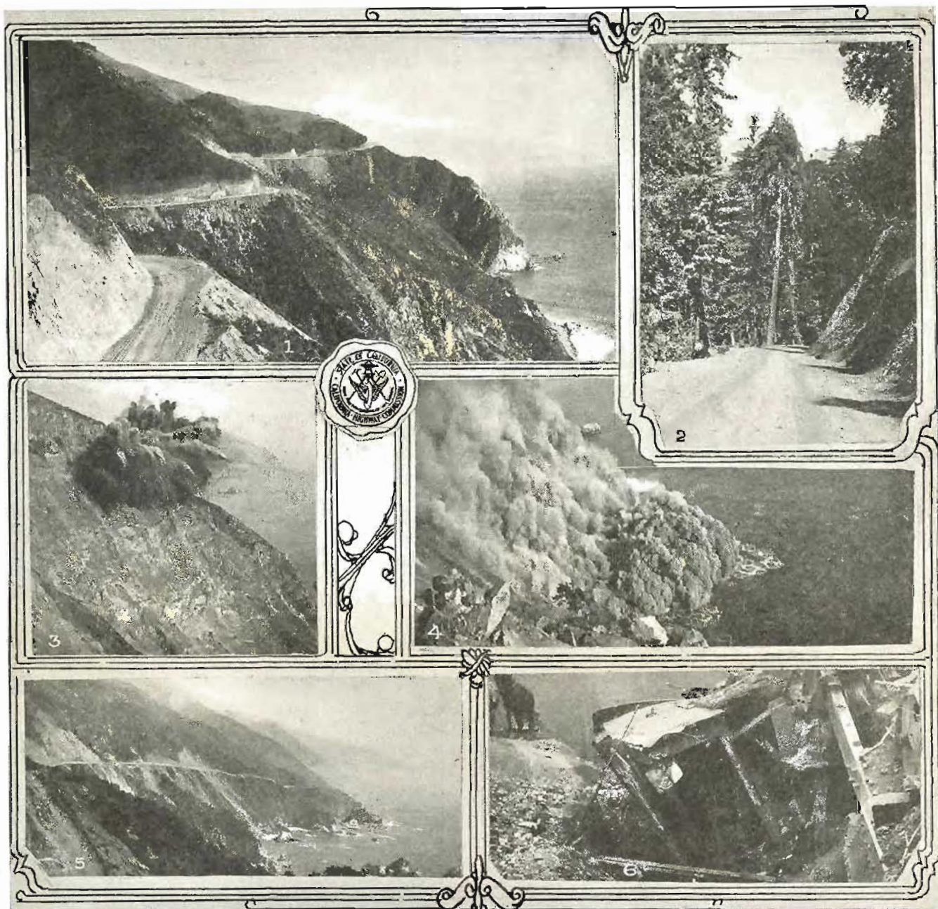
THE POLLOCK CONTRACT ON THE MONTEREY COAST—Views on the recently completed Pollock contract south of the Big Sur River, Carmel-San Simeon highway, Monterey County; (1) the completed grade high above the breakers of the Pacific; (2) Redwoods near the Big Sur; (3) a blast at Grimes Point; (4) the great cloud of dust and rock settling over the ocean; (5) another view of the completed grade and the Coast line below; (6) troubles of the contractor, a power shovel wrecked by a slide. (Division V.)
