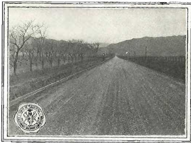
NEW SECTION OF TAHOE-UKIAH ROUTE—Graded and surfaced highway west of Williams, Colusa County, Division III.
