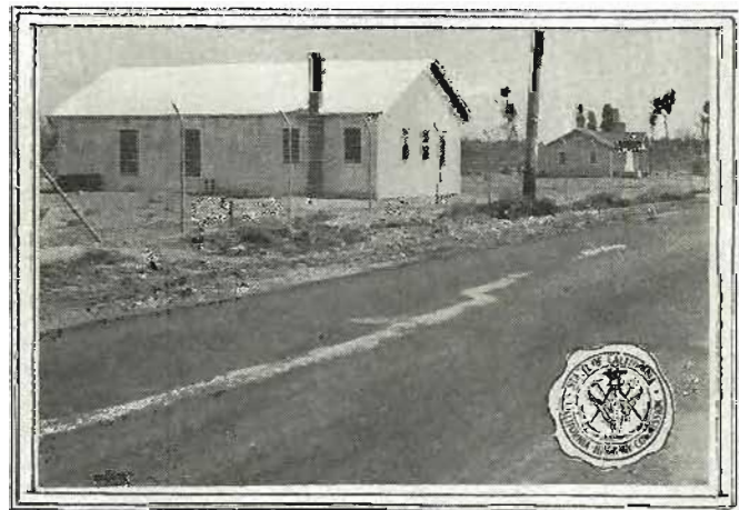
NEW MAINTENANCE STATION—Foreman's cottage and warehouse for equipment near El Rio, Ventura County, Division VII.
