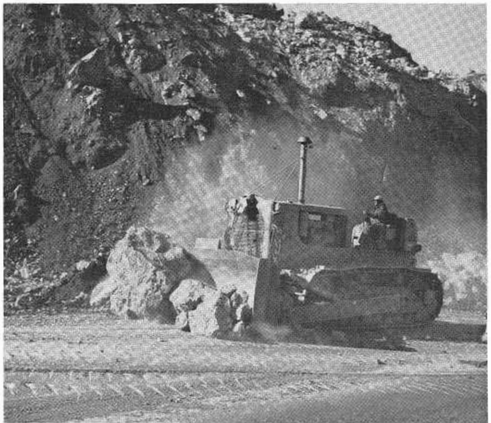
UPPER—Section of a cut taken just after a blast. The larger boulders will have to undergo secondary blasting operations before they can be hauled away. LOWER—A tractor clears boulders from the roadway shortly after a blast.
