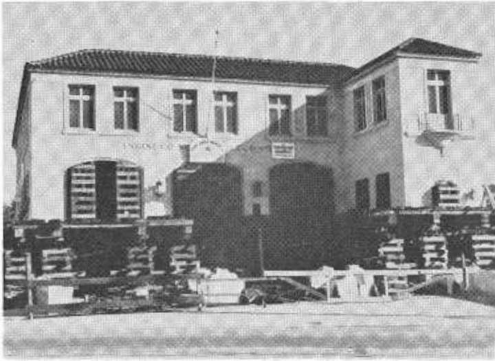
A fire station in the City of Los Angeles is relocated to clear right-of-way for the Hollywood Freeway. LEFT—Shows the building blocked up just before being moved. RIGHT—Shows the same building after it had been re-established and placed in use by the Los Angeles Fire Department in its new location.
