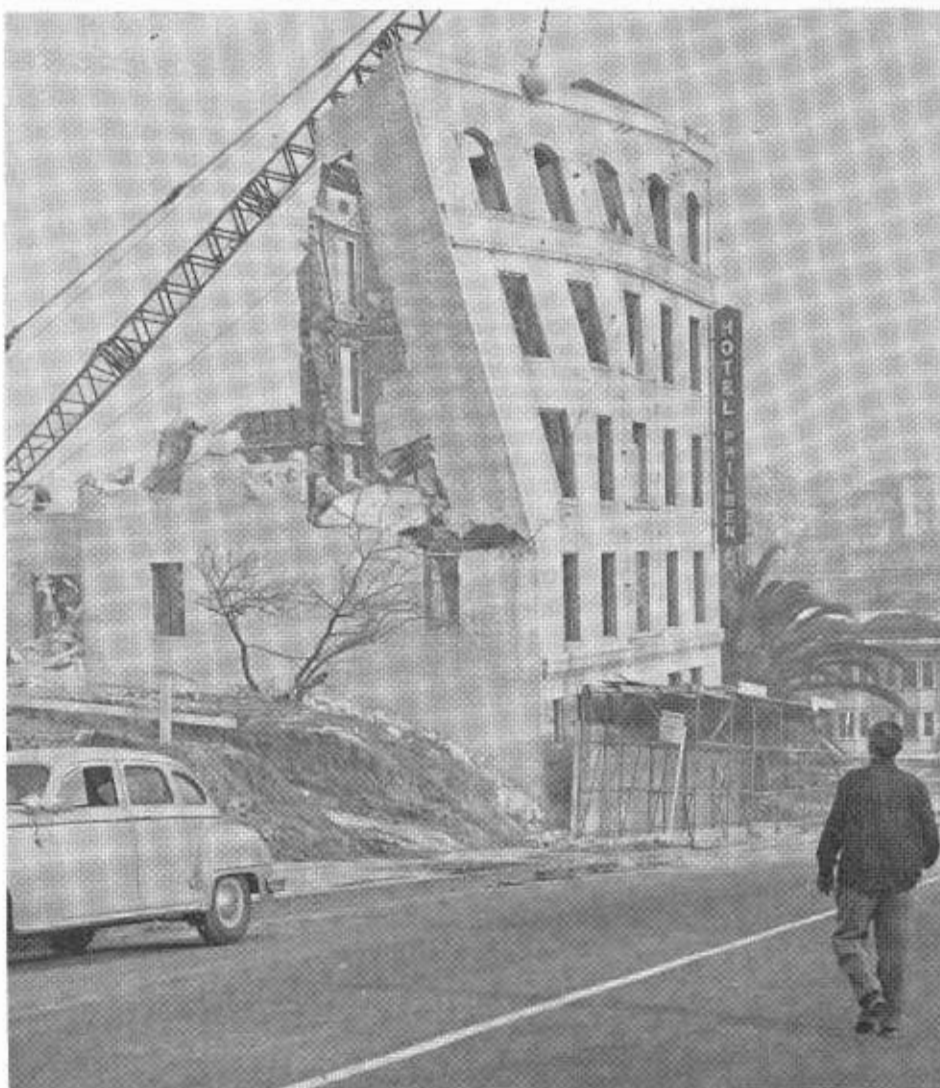
A 3,700-pound weight on the end of a long crane boom demolishes a concrete building to make way for a new freeway through downtown Los Angeles
