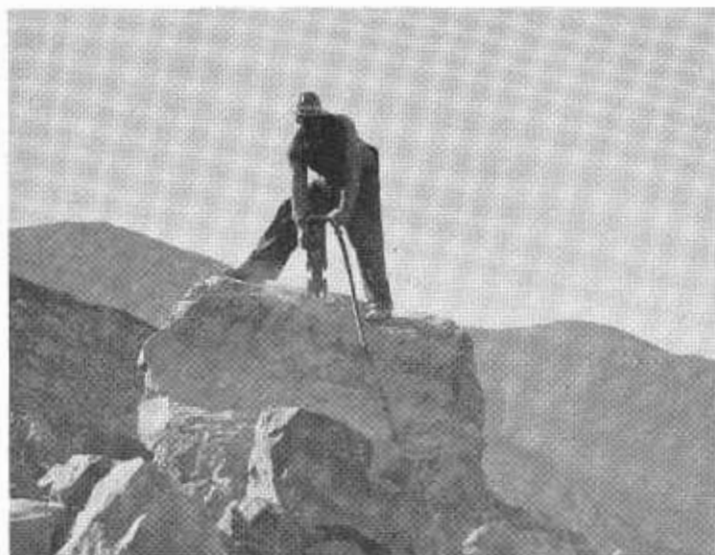
LEFT—A drill operator works away at a large rock left over from primary blasting in order to reduce it to pieces small enough for equipment to handle. RIGHT—A crew is engaged in secondary blasting operations on a rock not broken up small enough by the primary blast.
