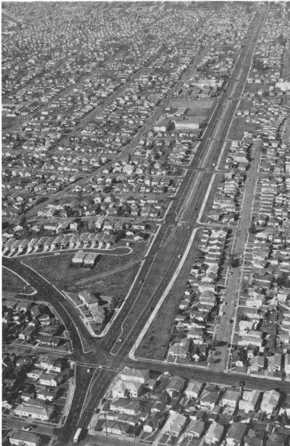
An aerial view of the recently completed Bancroft Avenue Freeway in Oakland. A noncontinuous street and railroad right-of-way was converted to a major thoroughfare and railroad parkway.
