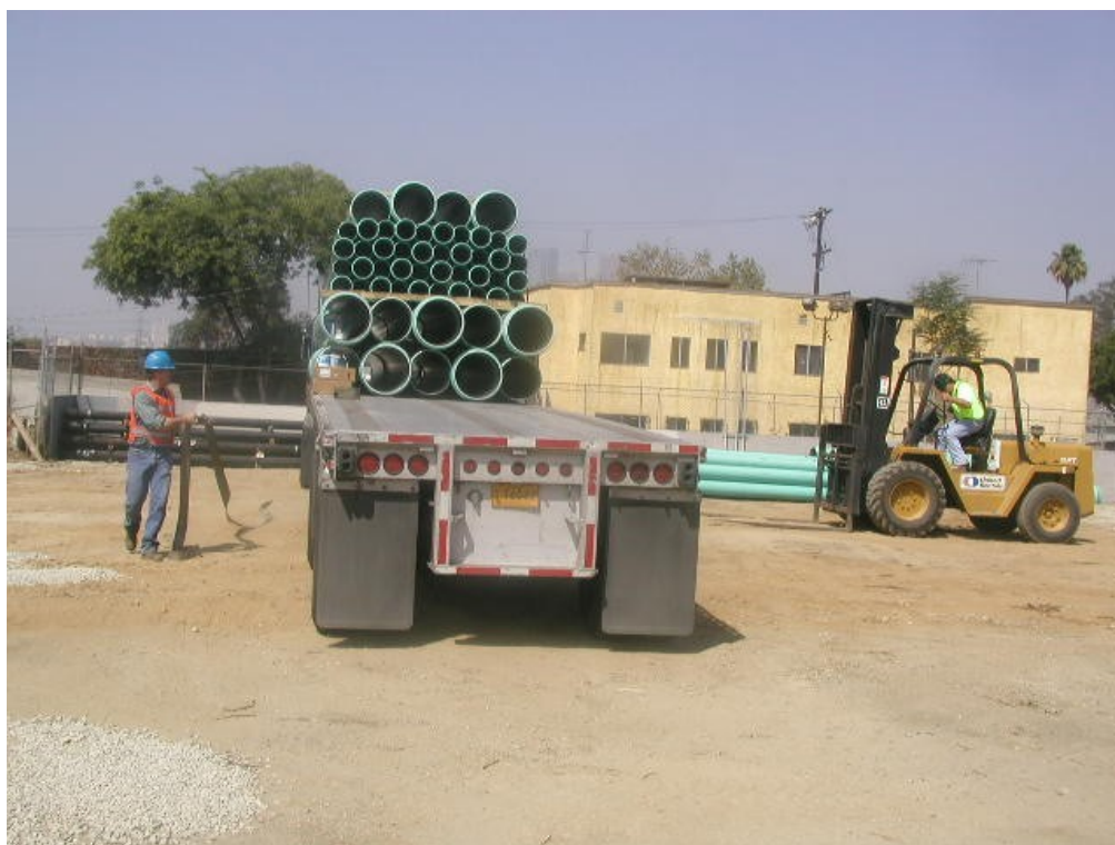
Unloading PVC storm drain piping.
