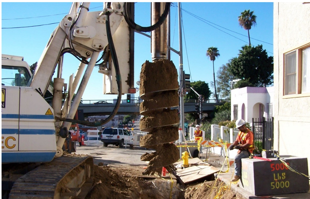
Drilling piles north side of Boyle Street.
