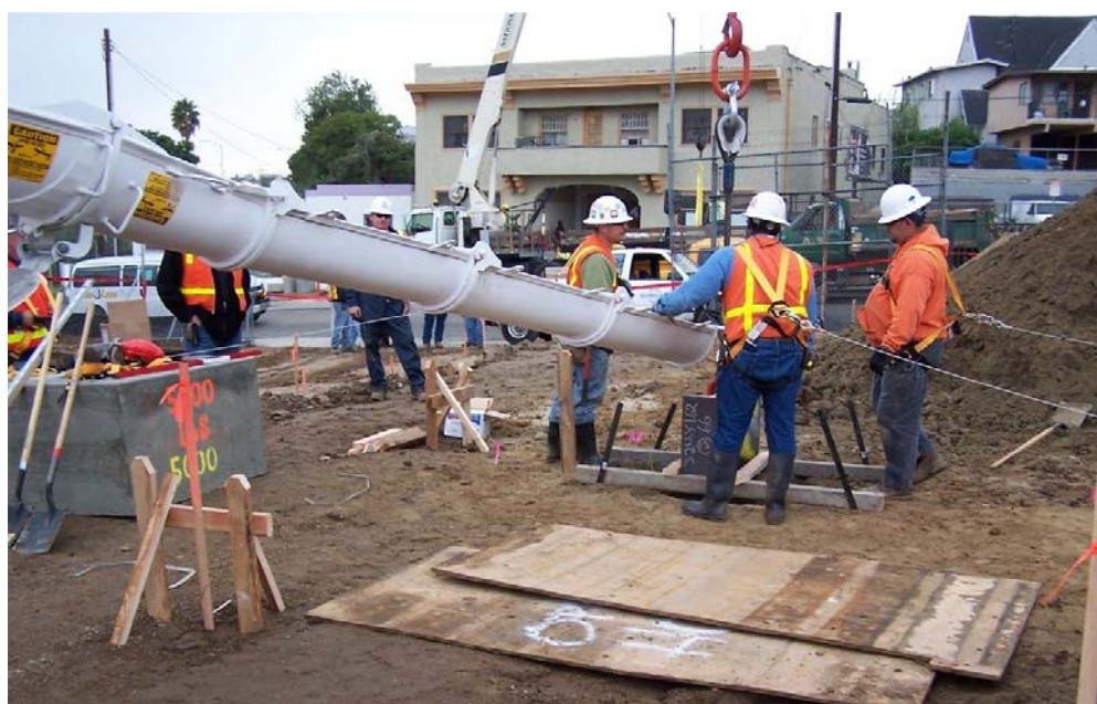
Slurry pile placement at Boyle.
