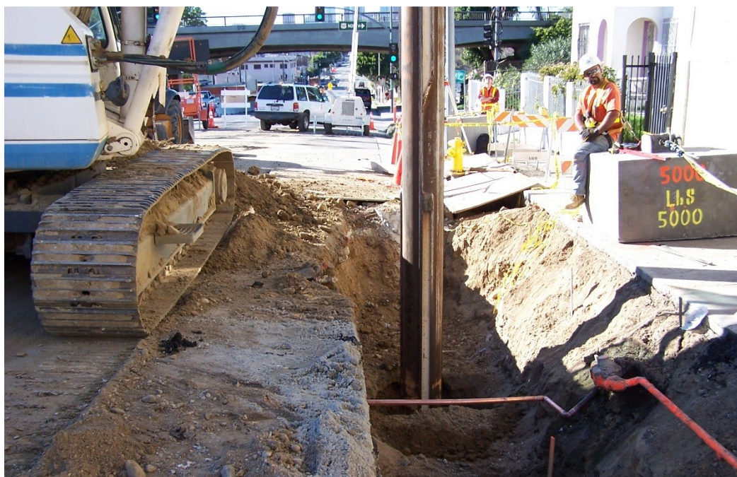
Drilling pile at Boyle.
