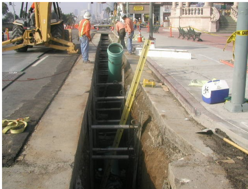
Placement of 18" storm drainage line at 1 st and Boyle Avenue.
