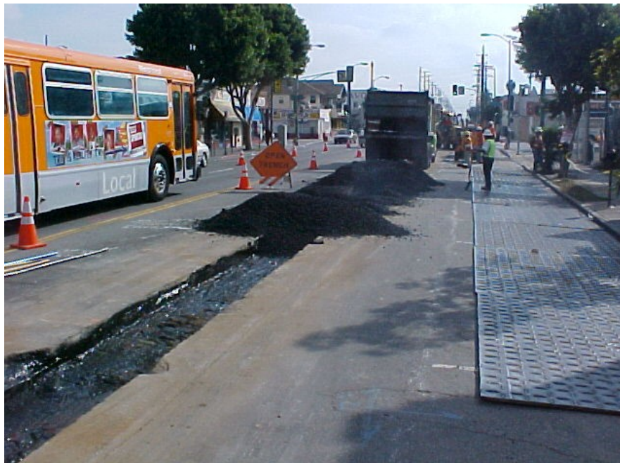
Repair of 1st Street after relocation of 12" water line.
