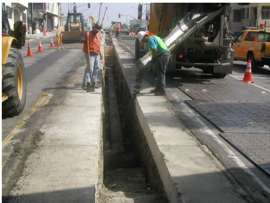
Placement of slurry over 12-inch water line.
