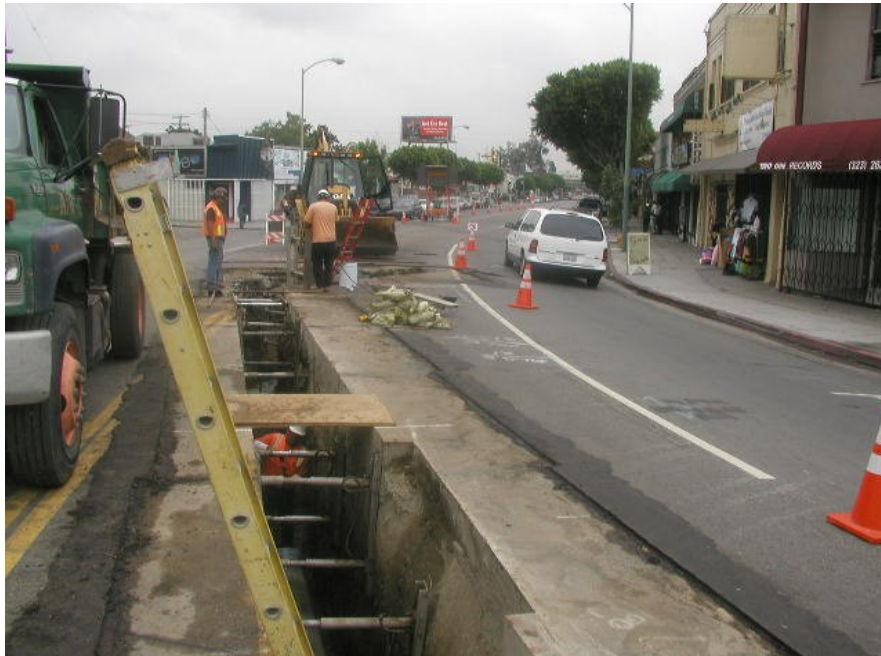
Placement of 12-inch water line along 1 st Street.
