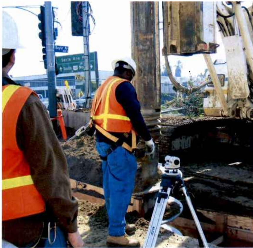
Drilling shaft in preparation of soldier pile placement at 1 st Street and Boyle Avenue.
