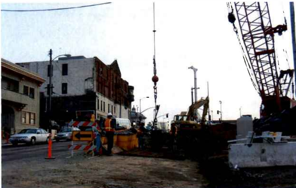
Soldier pile installation at Boyle Station.
