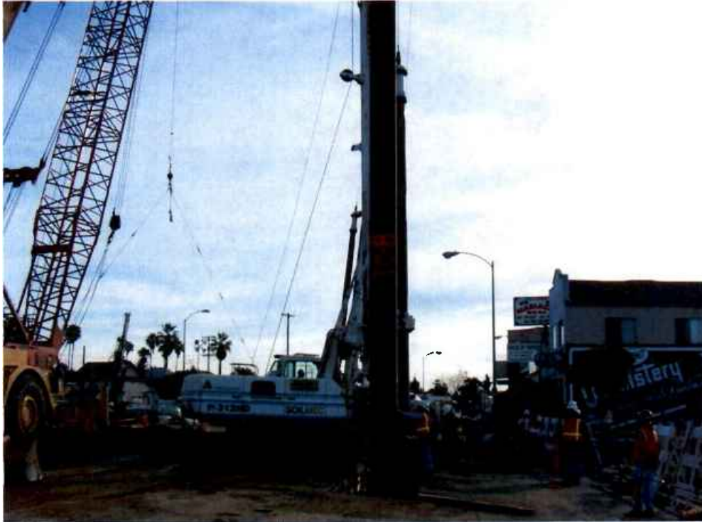
Soldier pile installation at Boyle Station.
