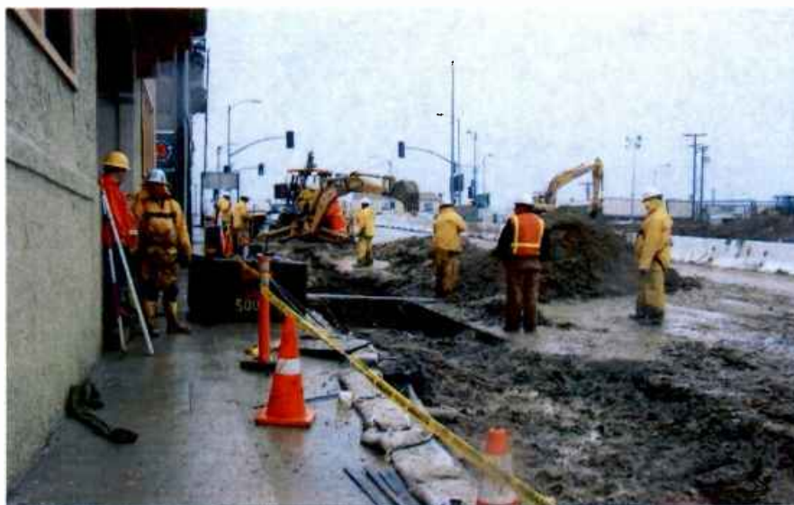
Trenching along 1 st Street in preparation of soldier pile installation.
