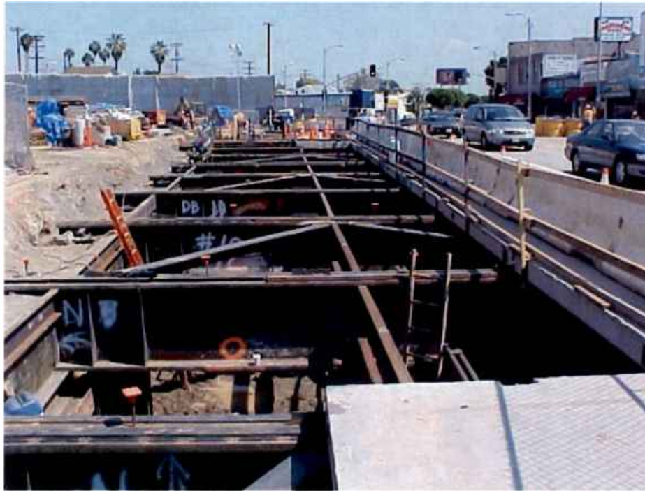
Deck beams and temporary street decking at Boyle Station.
