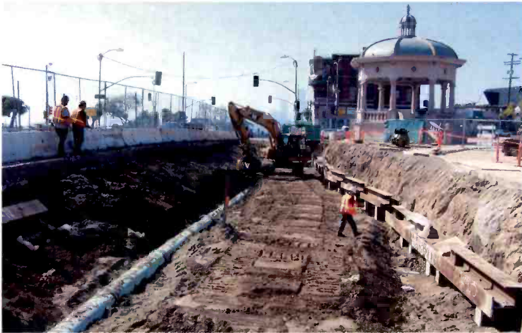
Preparatory excavation work prior to deck beam and temporary street decking installation at Boyle Station.
