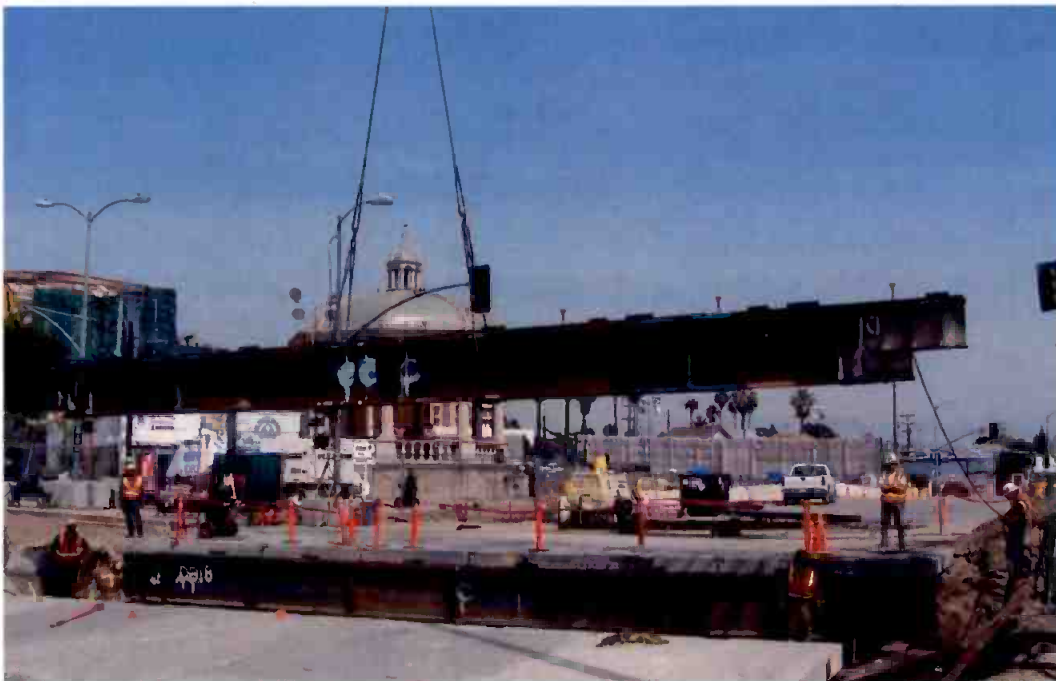
Deck beam being placed at Boyle Station.
