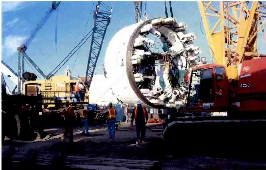
Assembly of Tunnel Boring Machines.
