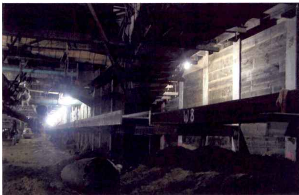
Soto Station structural excavation.
