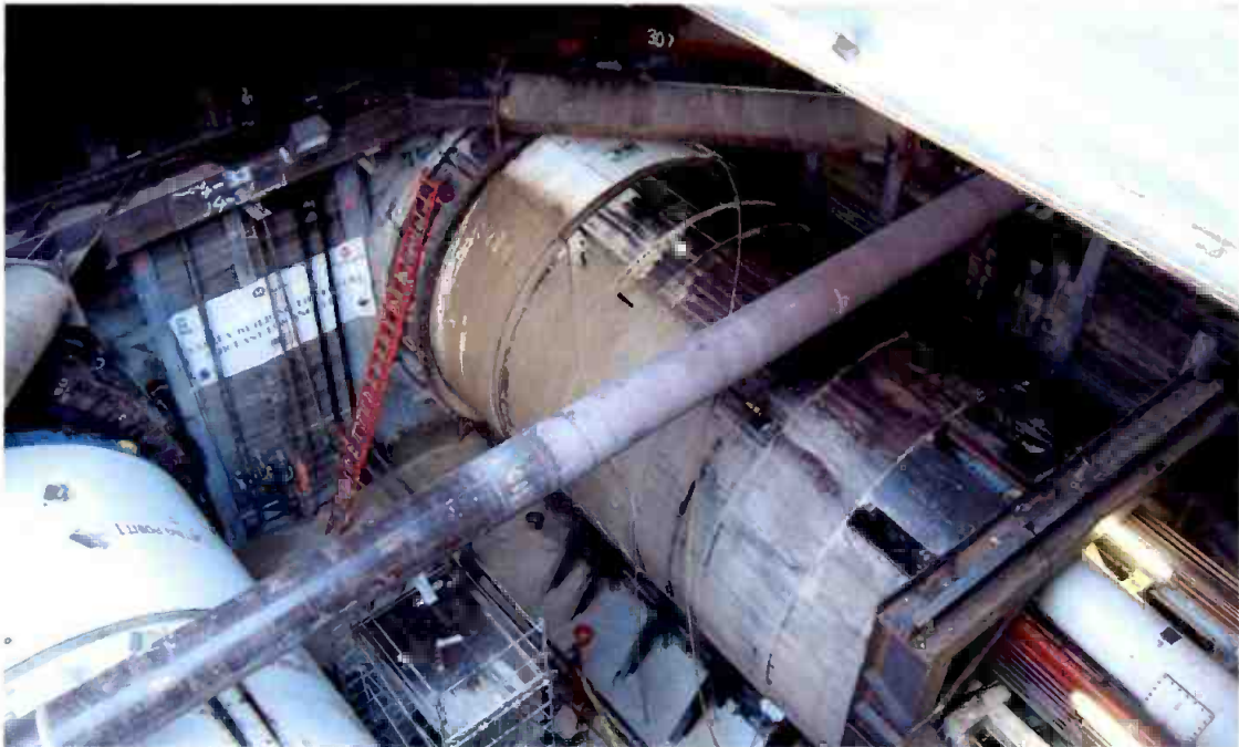
Eastbound Tunnel Boring Machine in operation.
