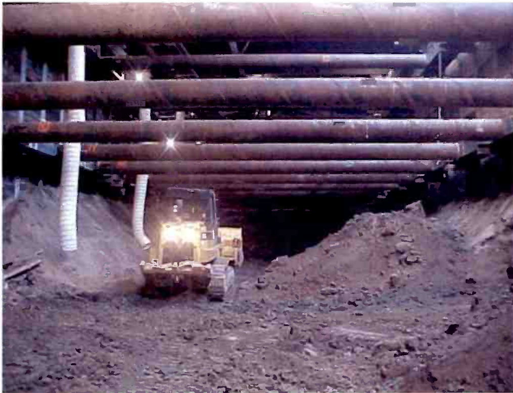
Soto Station structural excavation.
