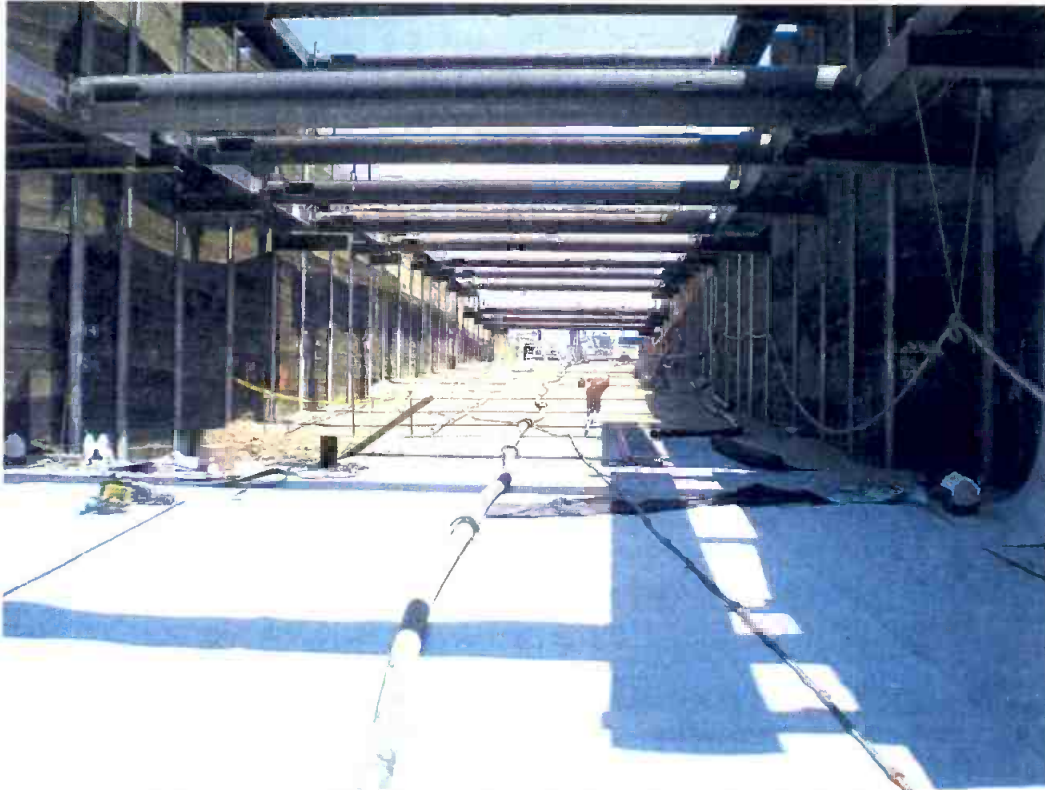
Preparation for the mud mat slab at the East Portal.
