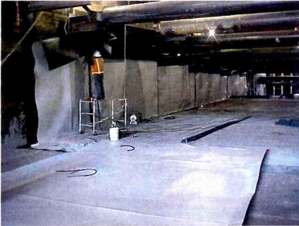
HDPE placement at the West Portal.
