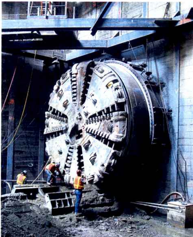
Eastbound Tunnel Boring Machine arrival at Soto Station.
