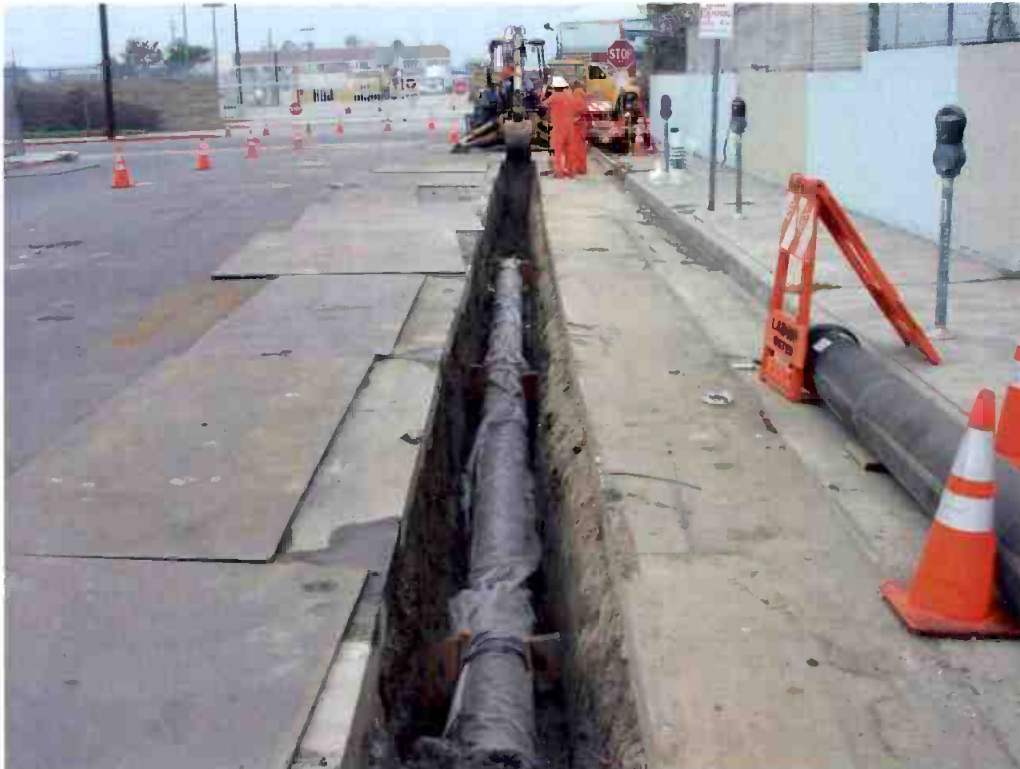
Segment 1 waterline relocation.
