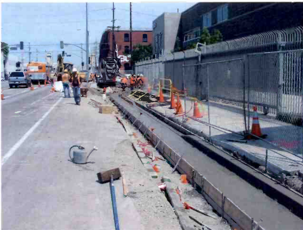
Segment 2A new curb and gutter.
