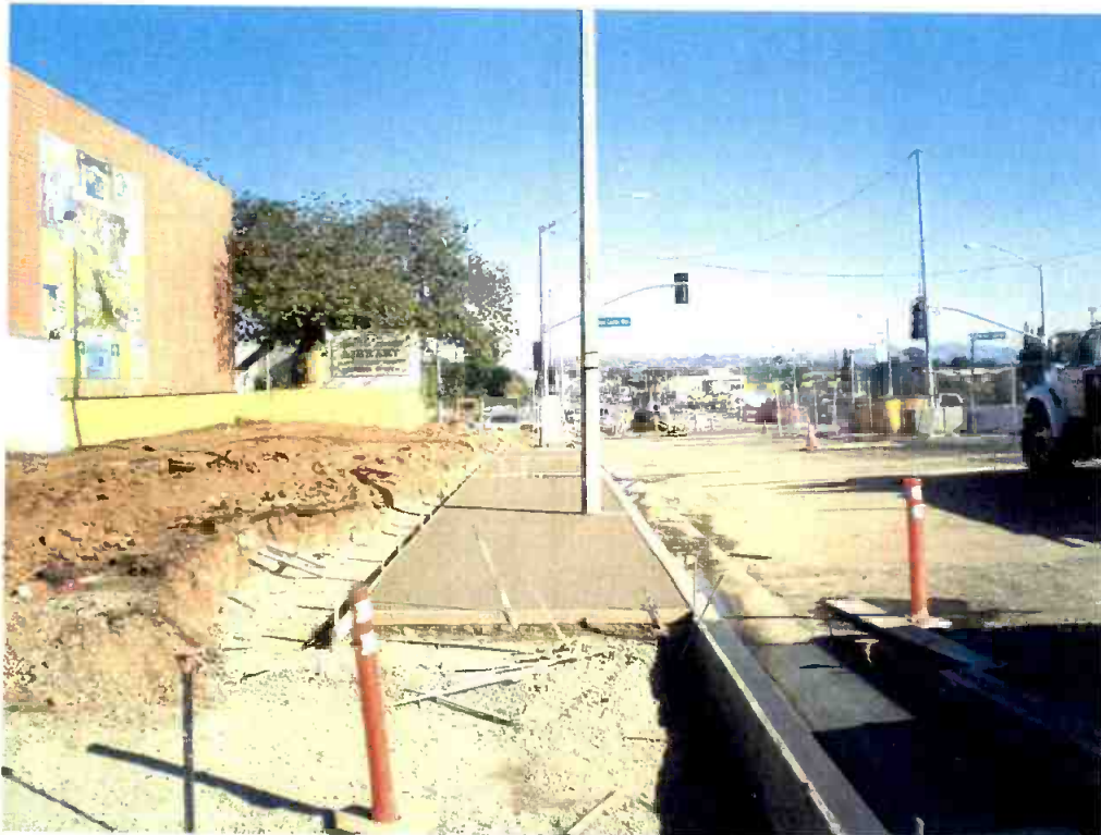
New curb and sidewalk construction within Civil Segment 7.
