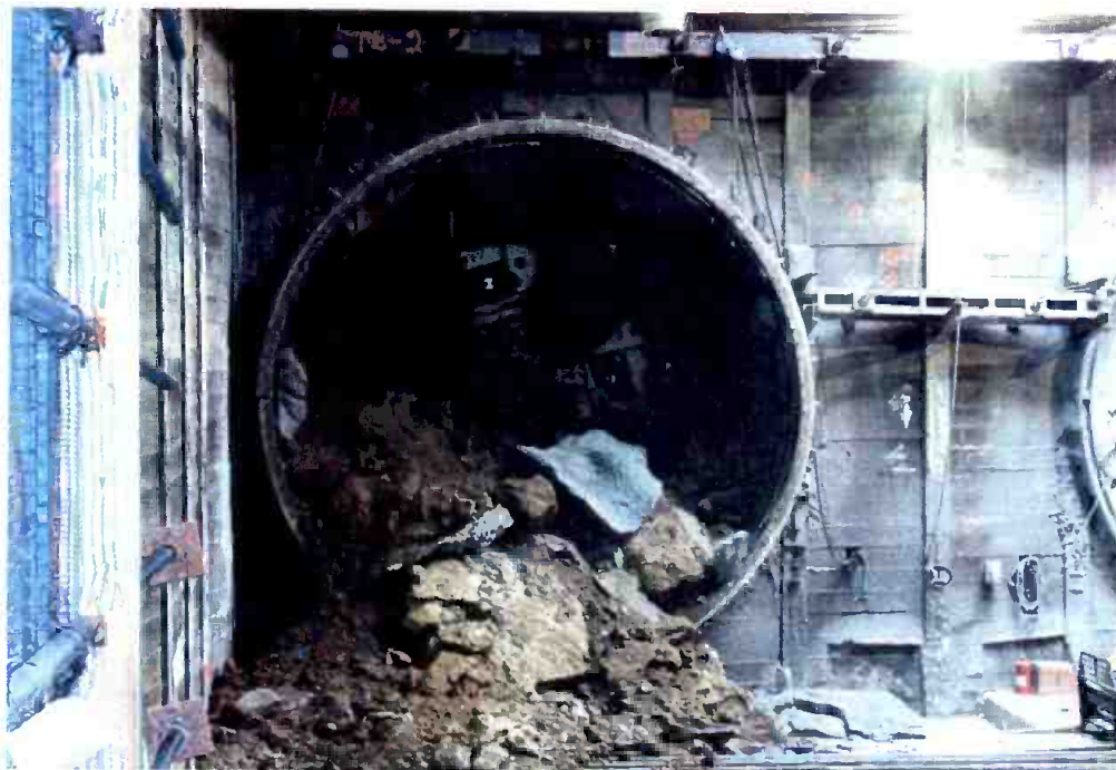
Eastbound EPBM breakthrough at East Portal.
