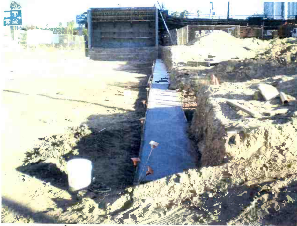
Construction of MSE wall Civil Segment 1.
