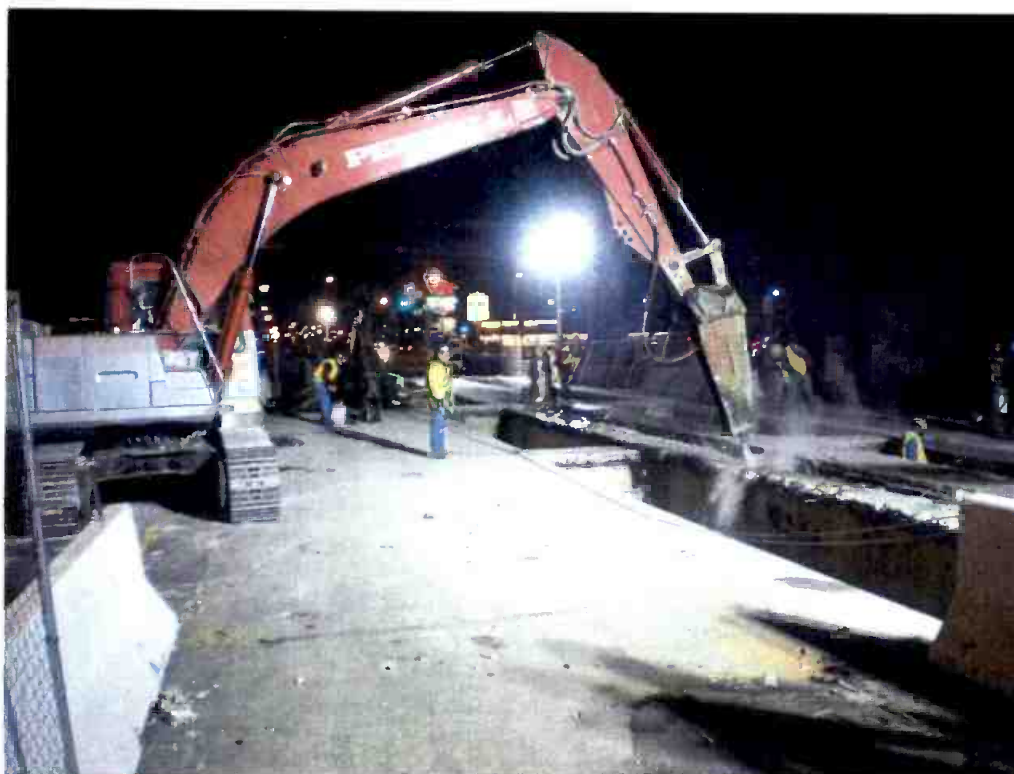
I-710 bridge demolition required for structural strengthening.
