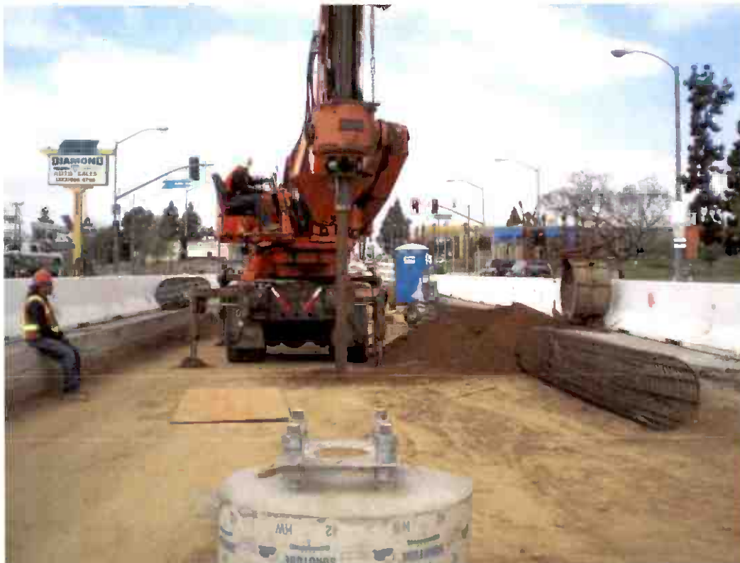
Placement of OCS pole foundations within Segment 7
