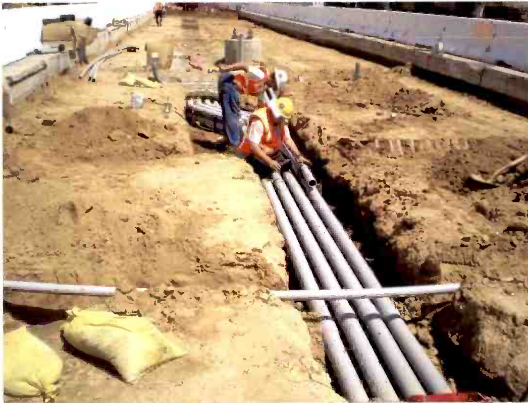
Placement of communications ductbank within Segment 7
