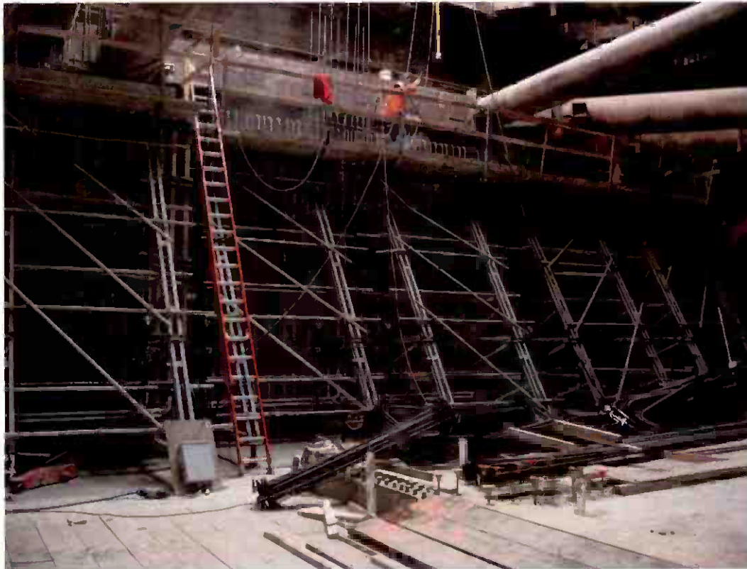
Boyle Heights/Mariachi Plaza Station north wall pour from track level to mezzanine level
