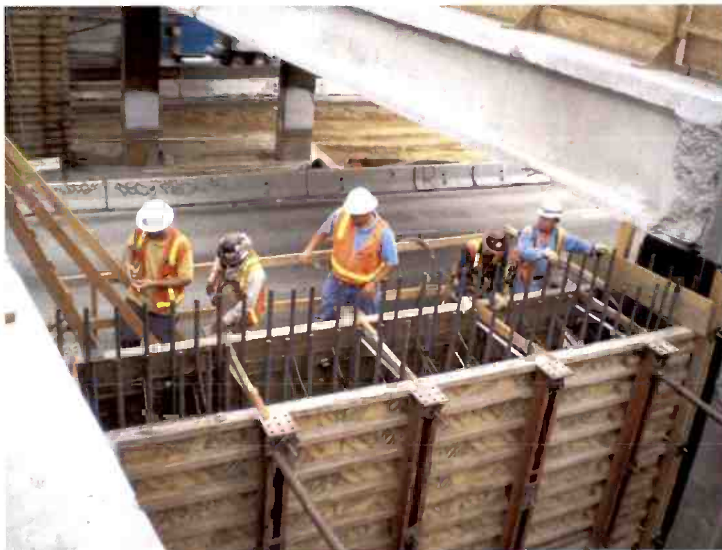
Preparing I-710 Freeway Bridge pier foundation for concrete placement
