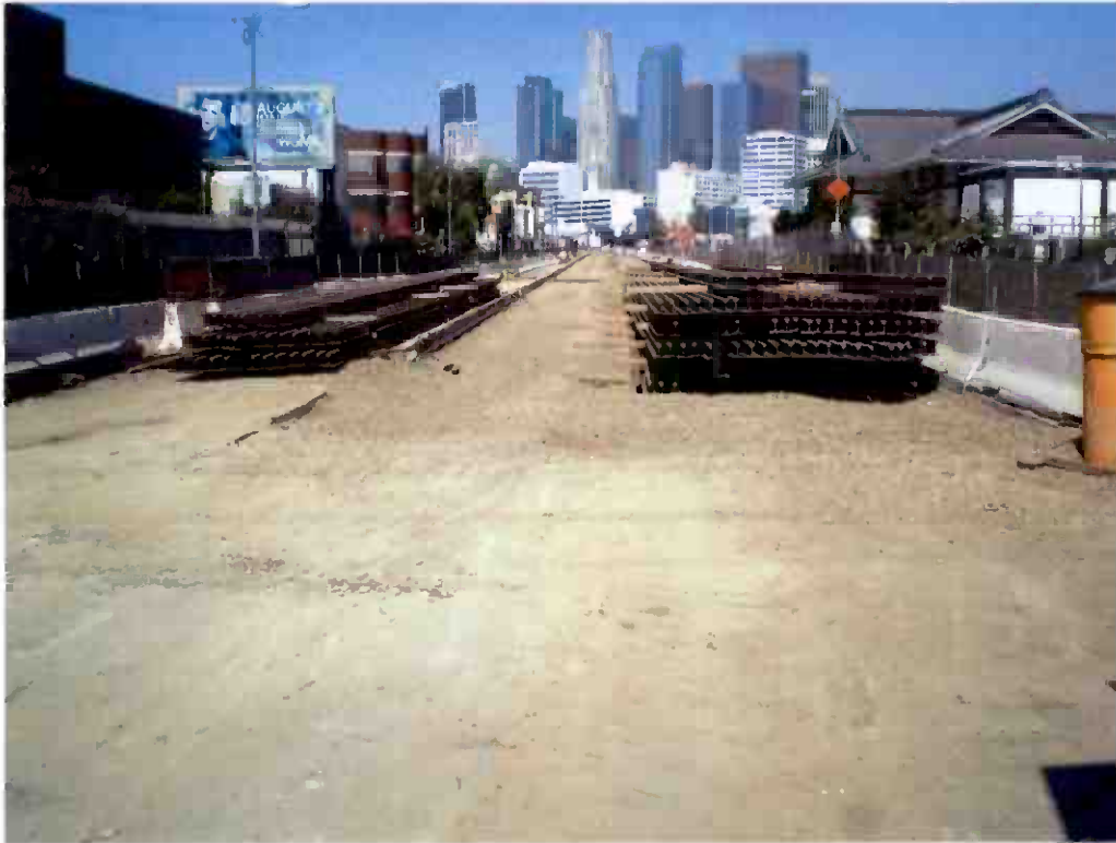
Track rail stockpiled within the LRT guideway – Civil Line Segment 2A.
