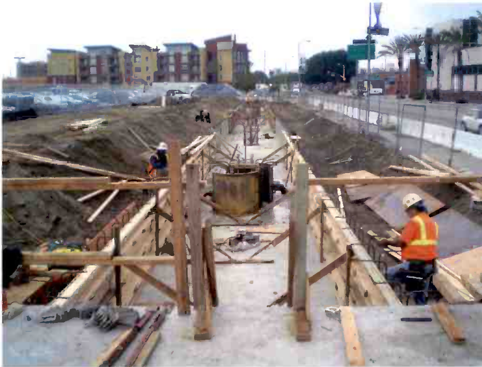
Placement of station platform forms for the Little Tokyo/Arts District Station.
