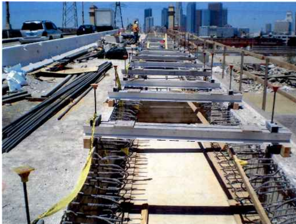
1st Street Bridge girder strengthening.
