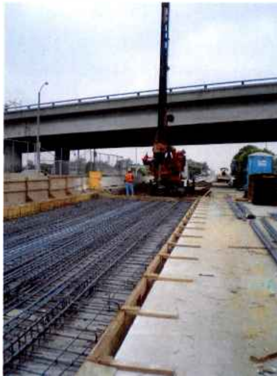
Construction of OCS pole foundations.
