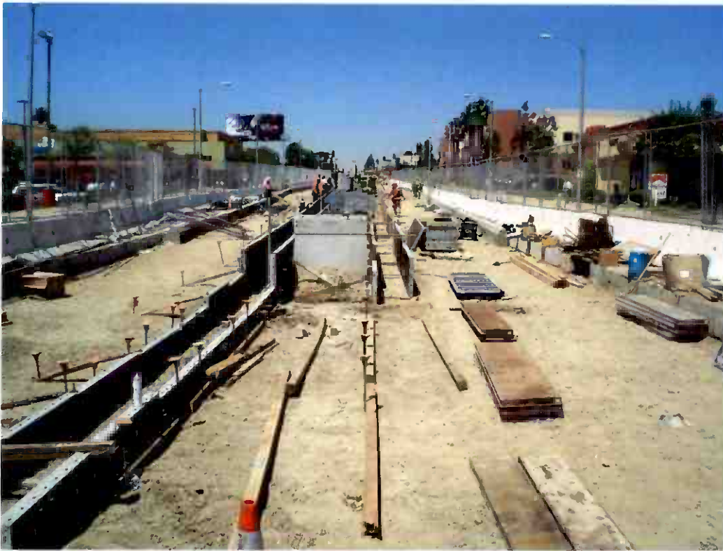
Construction of pedestrian access ramp at Atlantic Station.
