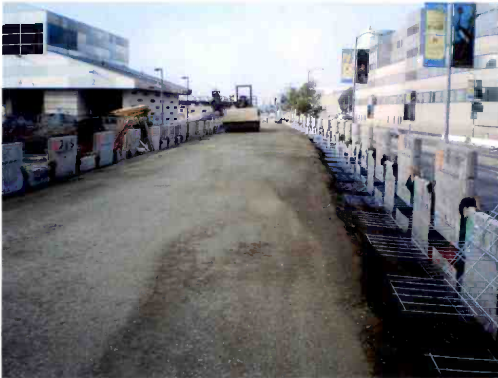
Construction of Mechanically Stabilized Earth (MSE) wall at the US 101 Freeway LRT Bridge.
