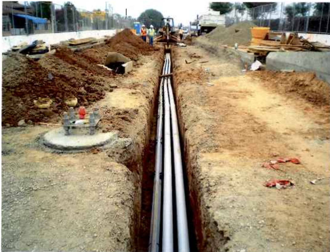
Ductbank installation along guideway within Segment 6.
