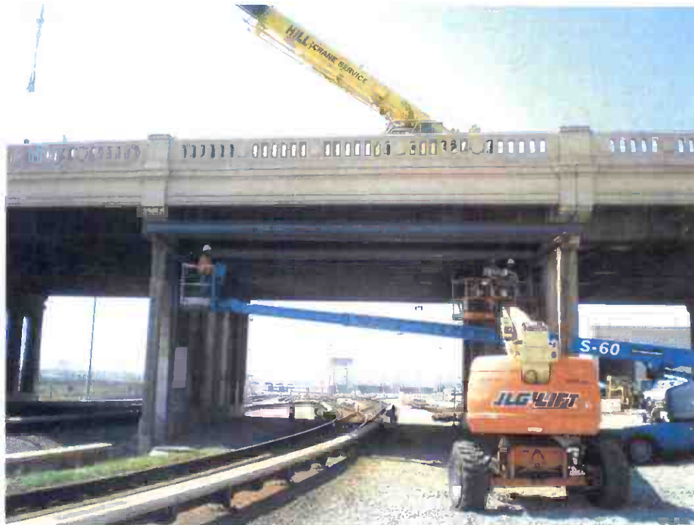
Installation of false work at the 1st Street Bridge.
