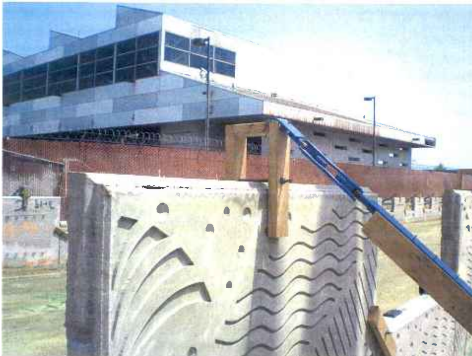
Placement of the MSE wall panels at the US 101 Freeway LRT Bridge Overcrossing.
