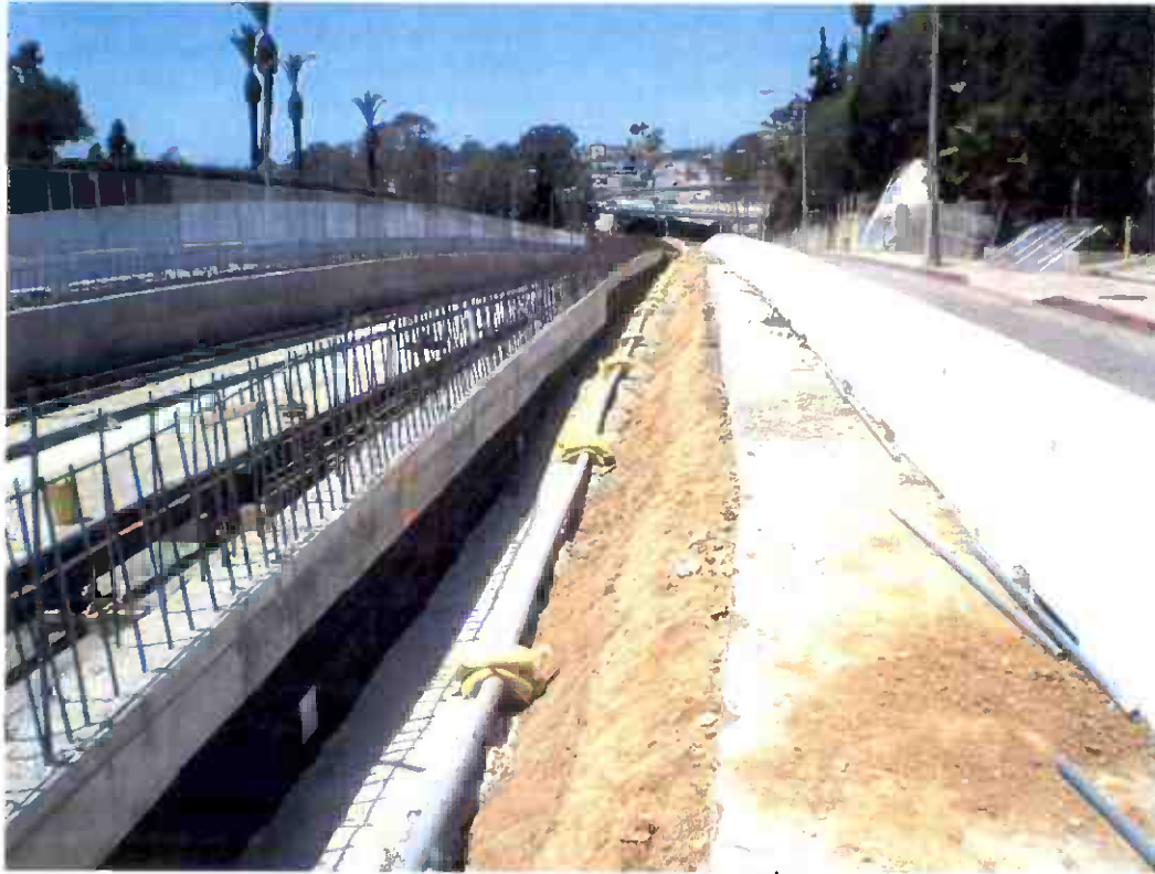
U-channel construction along 3 rd Street.
