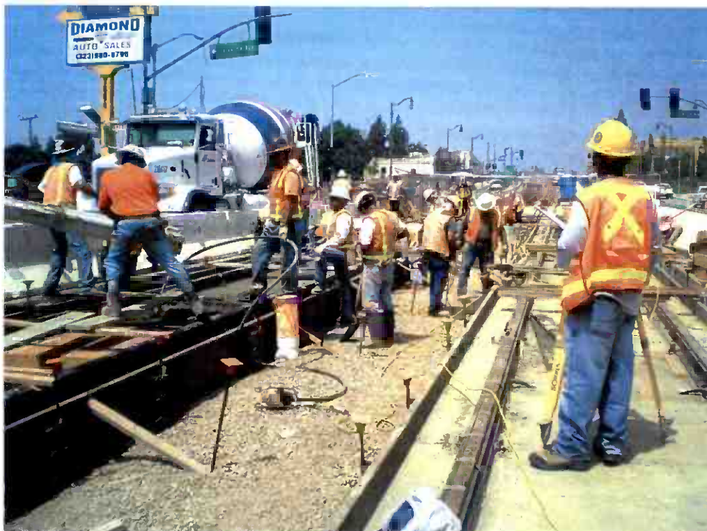
Placement of embedded trackwork at La Verne Avenue and 3 rd Street.
