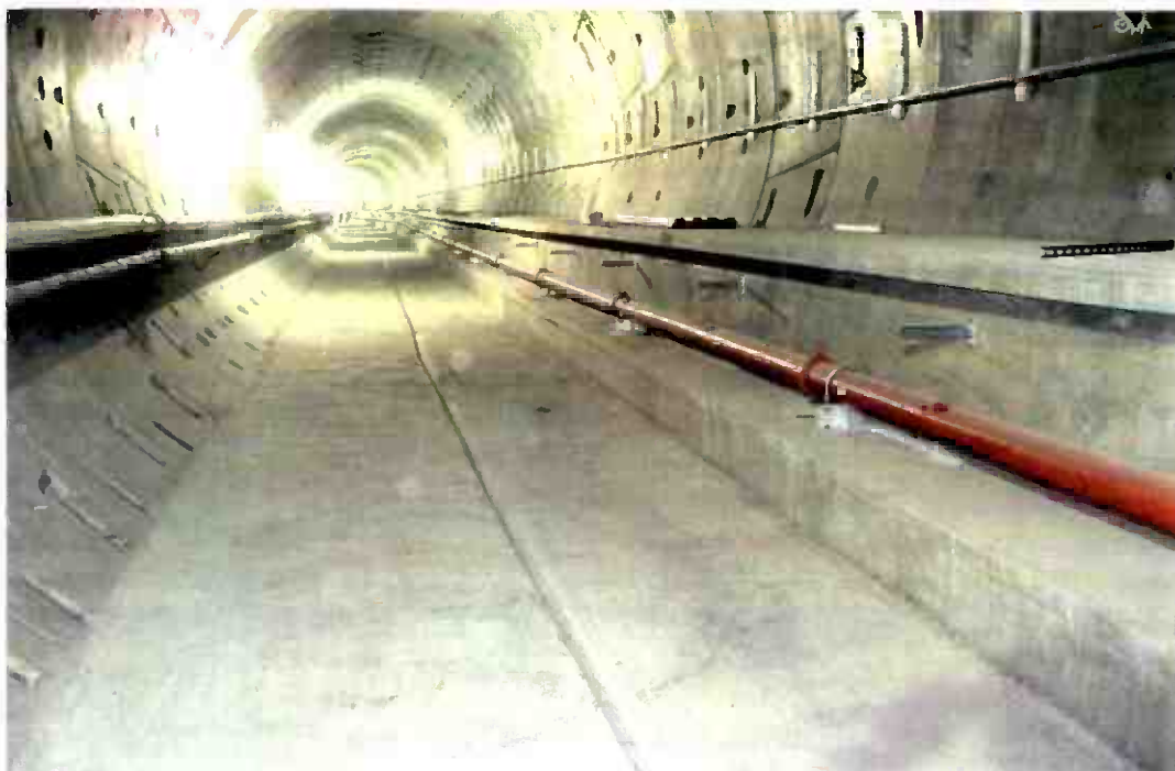
Construction of tunnel walkway.
