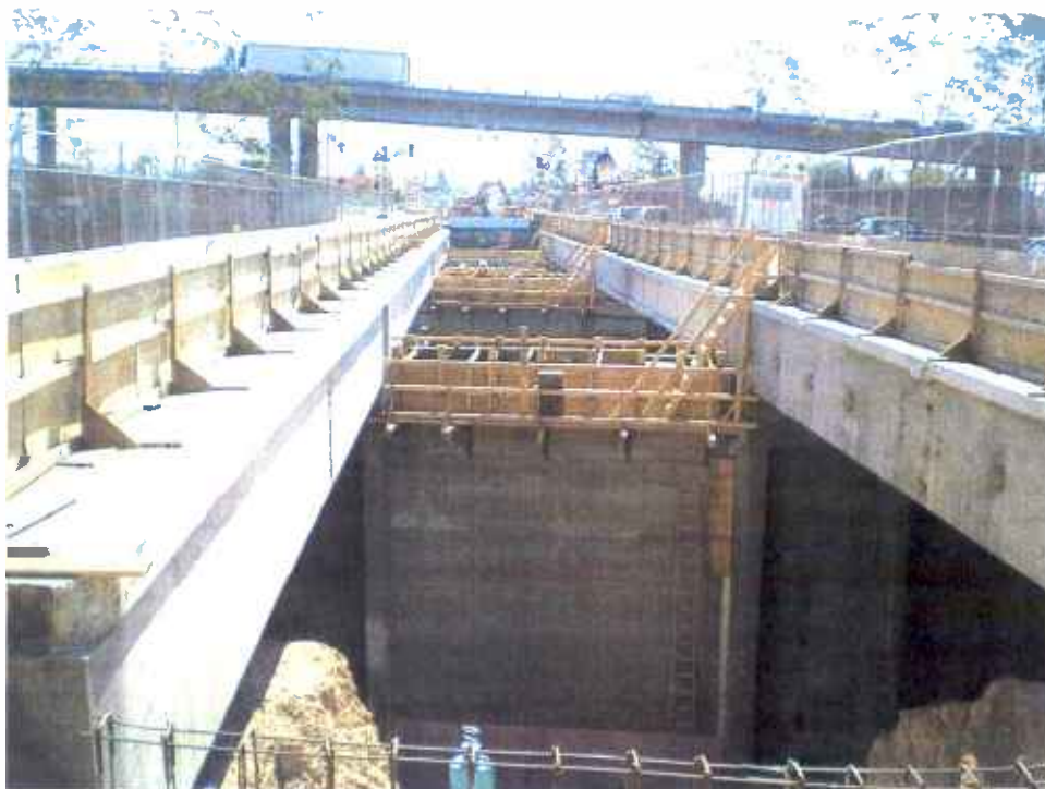
I-710 Freeway Bridge Overcrossing pier foundations.
