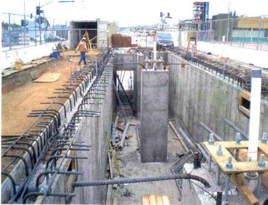
Construction of the train control room at the East LA Civic Center Station.
