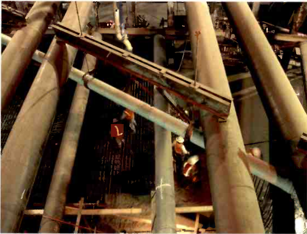
Placement of entrance invert slab concrete at Boyle Heights Mariachi Plaza Station.
