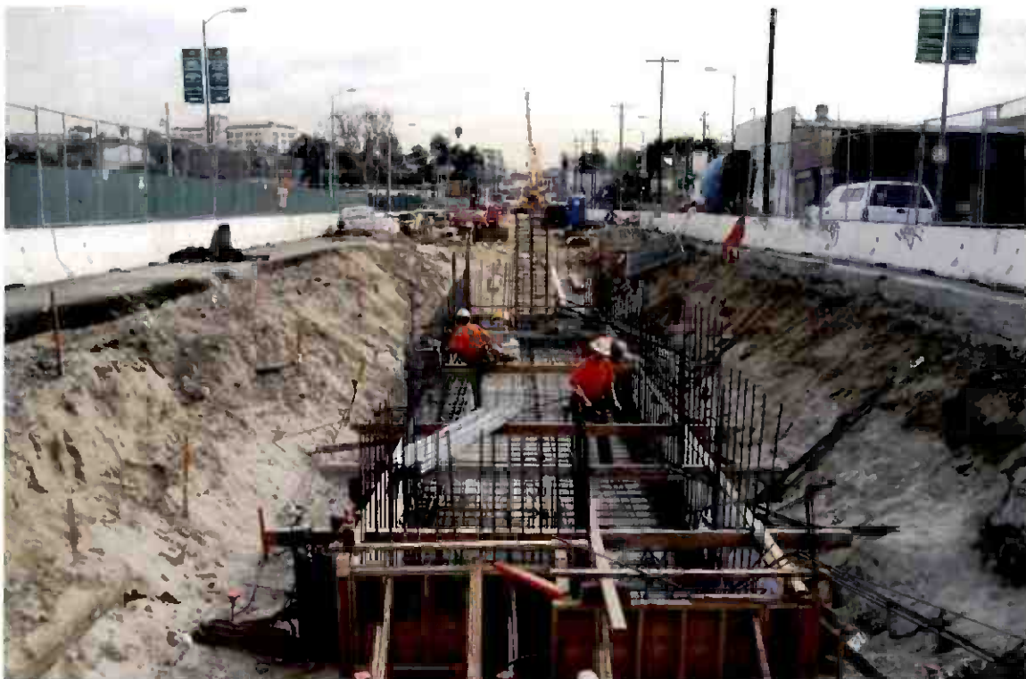
Pico/Aliso Station TCC room construction.
