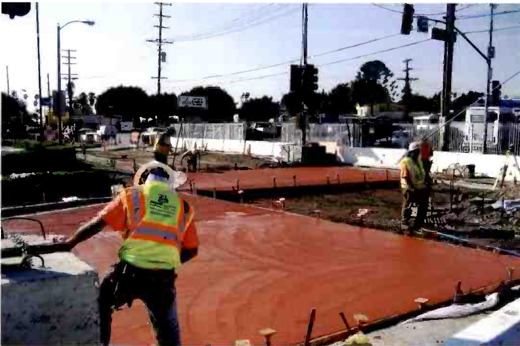
Construction of stamped colored pedestrian walkways at 3 rd and Indiana Streets
