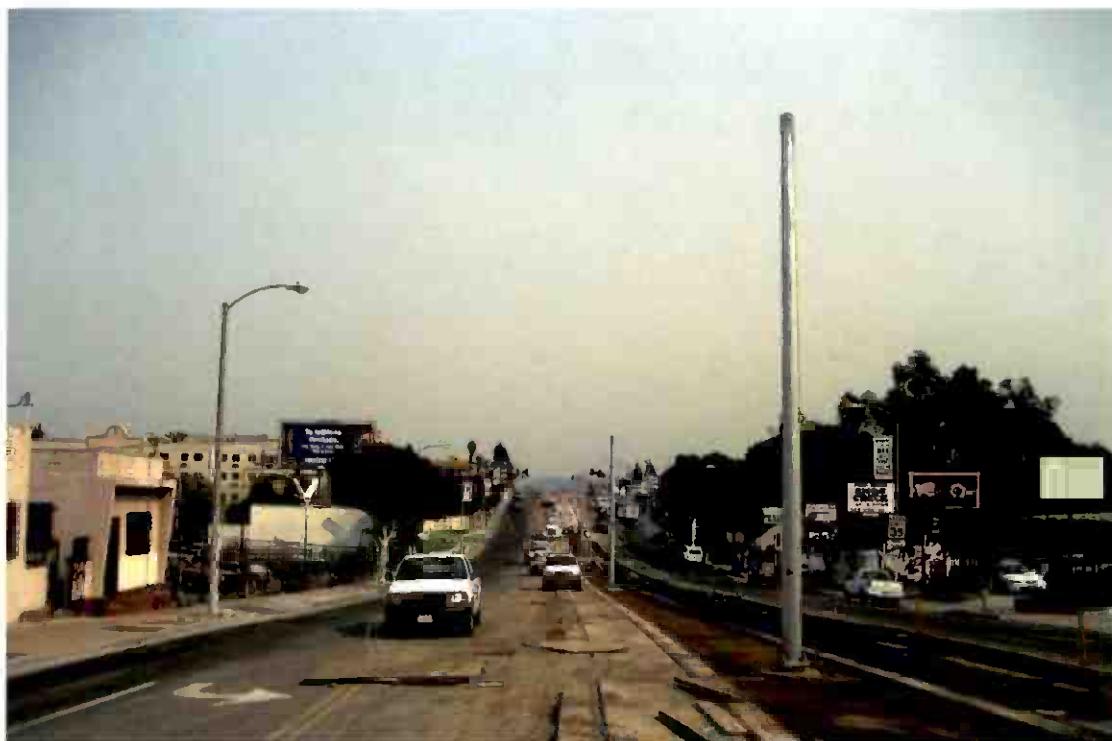
OCS pole installation within Civil Line Segment 6.
