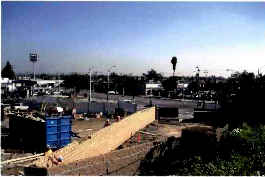
CMU wall construction for Traction Power Sub Station 6.
