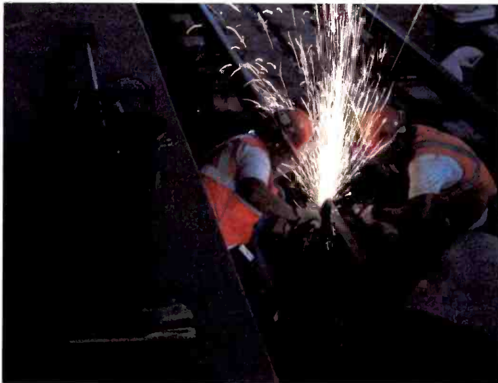
Welding rail within the tunnels.
