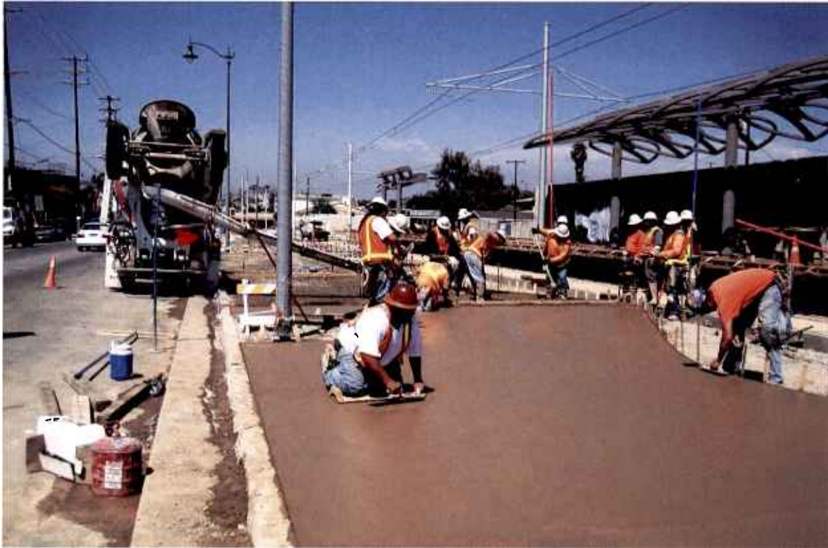
Placement of concrete walkways at Indiana Station.
