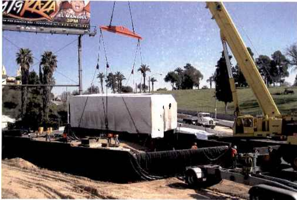
Lowering Traction Power Substation #4 on it's foundation.
