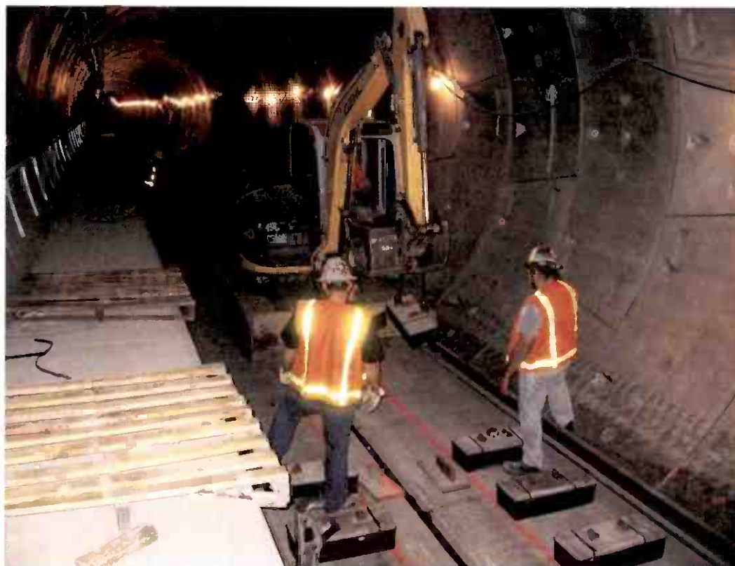
Placement of LVT blocks within the tunnels prior to rail installation.
