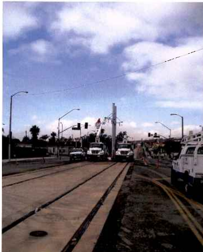
OCS hanger and wire installation within Segment 6.
