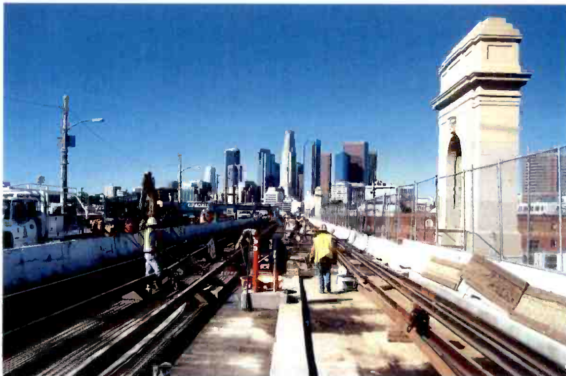
Track installation on 1 st Street Bridge.
