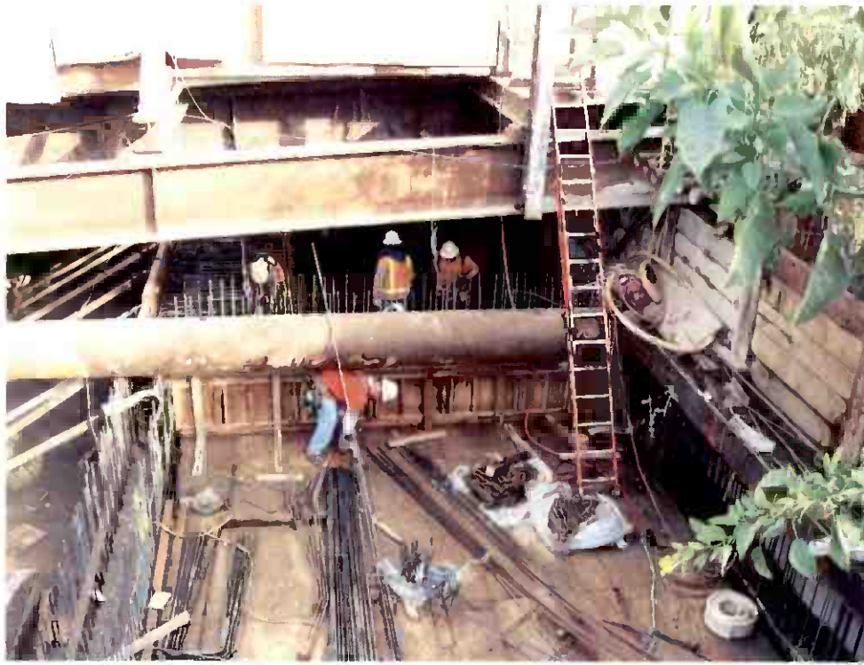
Roof rebar installation at the Boyle/Heights Mariachi Plaza Station.
