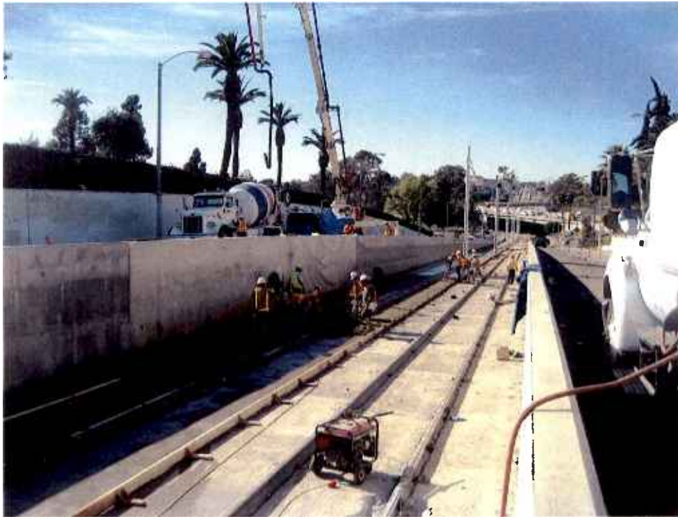
Eastbound guideway construction within the U-channel.
