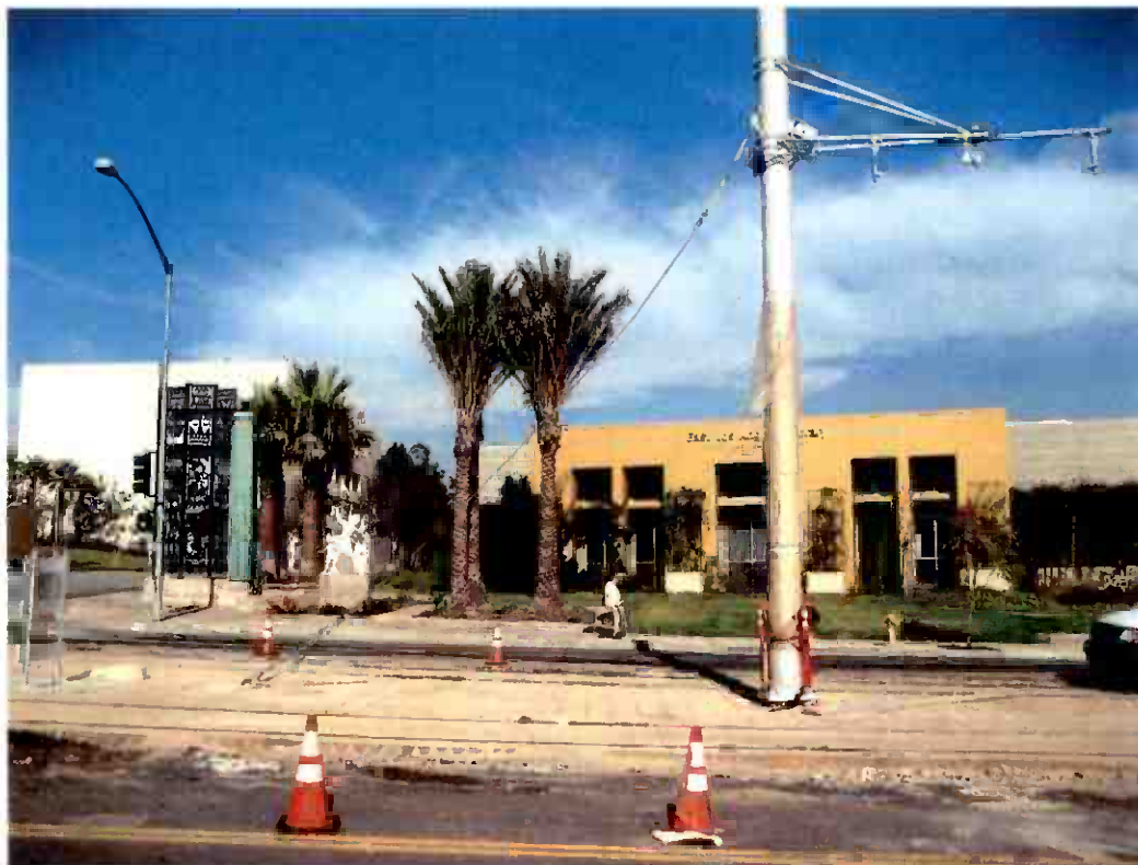
Segment 7 installation of OCS poles and hangers.
