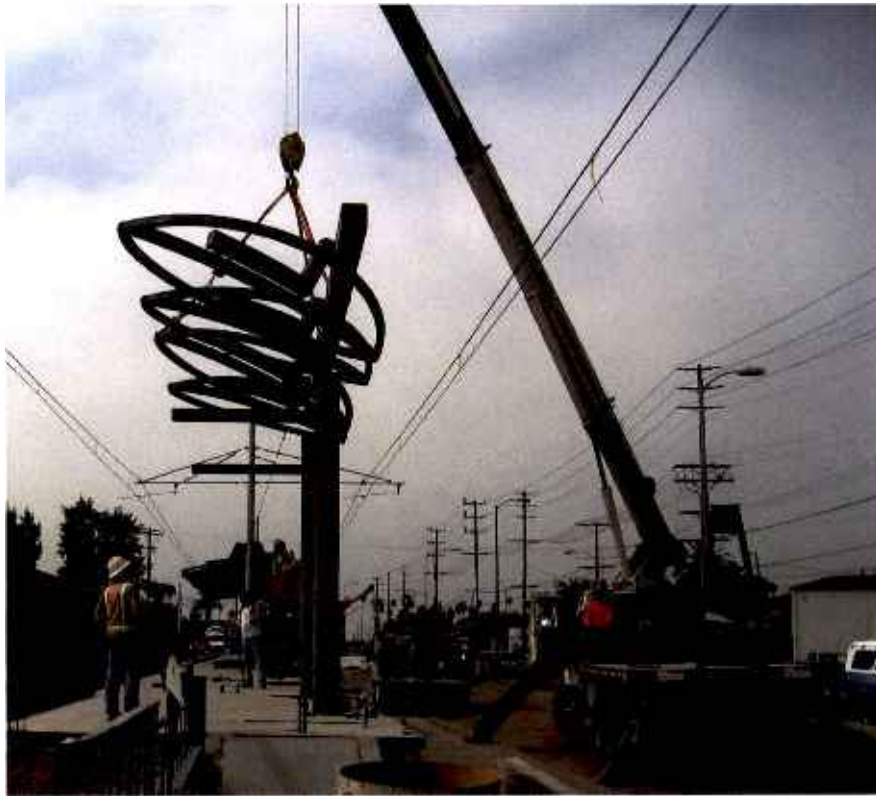
Installation of the canopy at Indiana Station.
