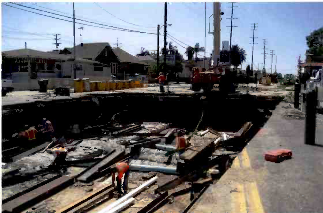
Removal of temporary street concrete deck panels at the East Portal.
