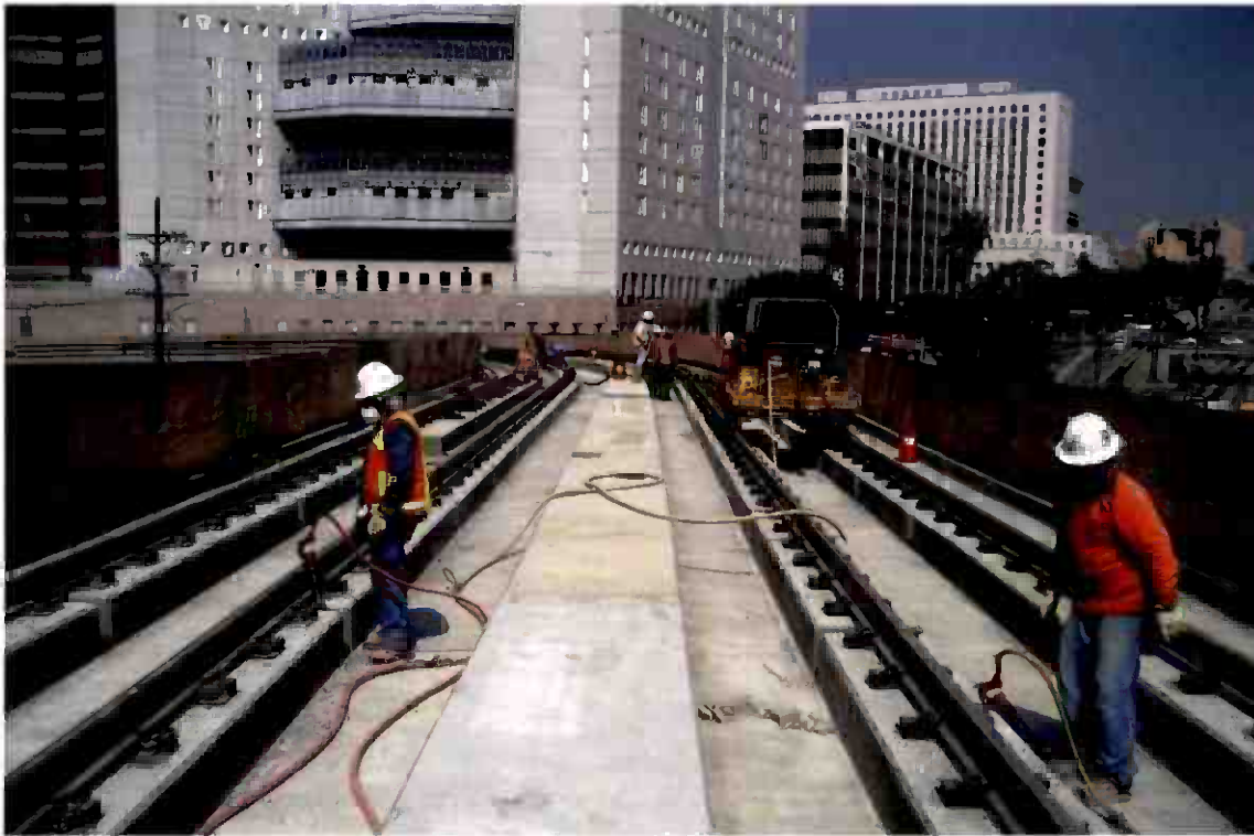
Rail installation on the US-101 Freeway Bridge LRT Overcrossing.
