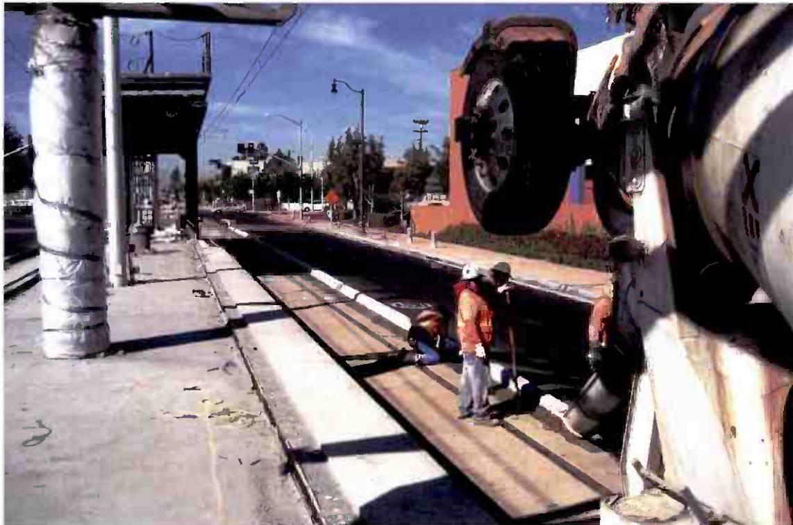
Placement of the street mountable curb on the westbound track guideway.
