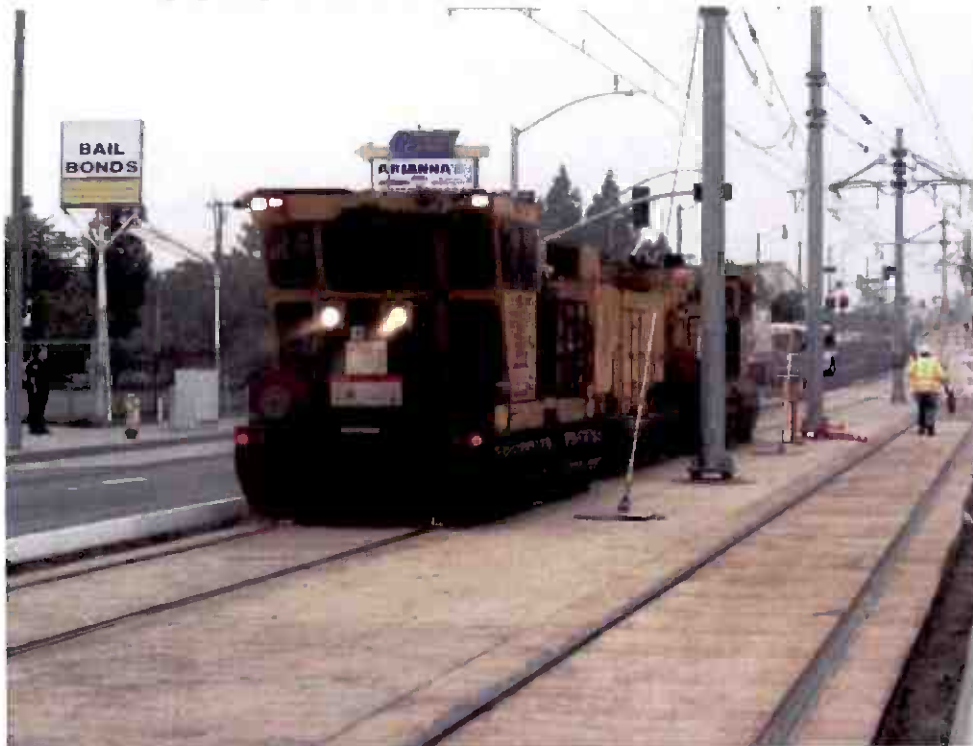
Rail grinding along the alignment, prior to rail vehicle testing.
