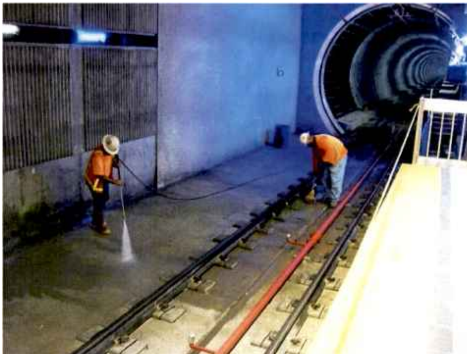
Final cleaning of track bed at Soto Station.
