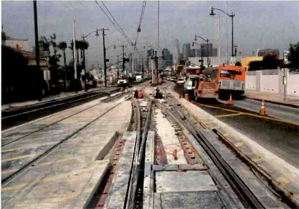
Crossover repair work at Clarence Street.
