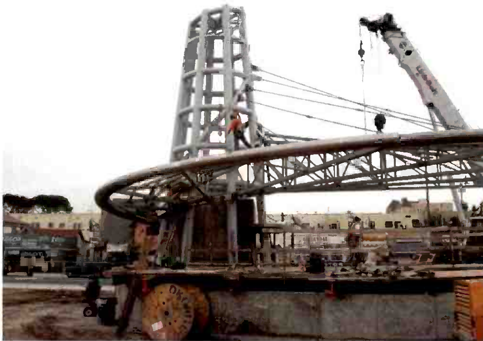
Installation of the Soto Station canopy at the pedestrian plaza level.
