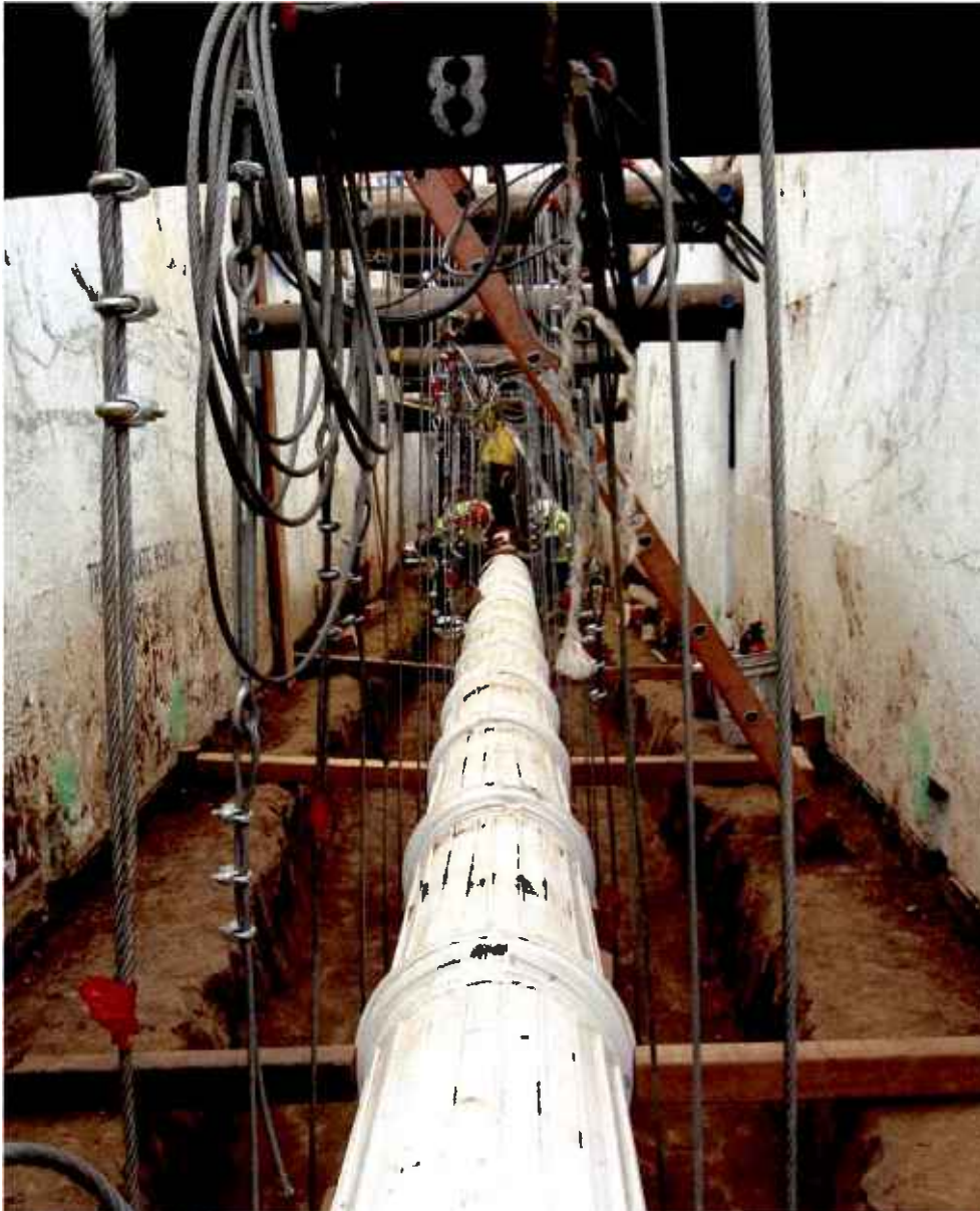
Encasement of existing sewer line prior to constructing the Pomona/Atlantic Parking Structure.
