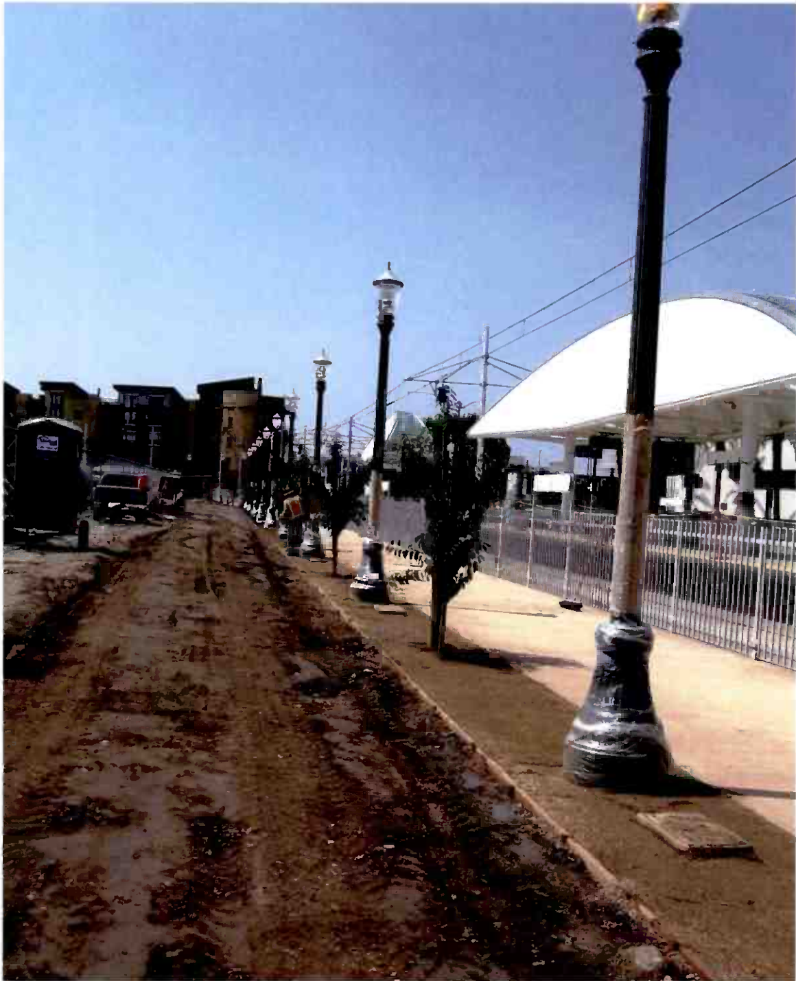
Installation of landscaping and pedestrian lighting at Little Tokyo/Arts District Station.
