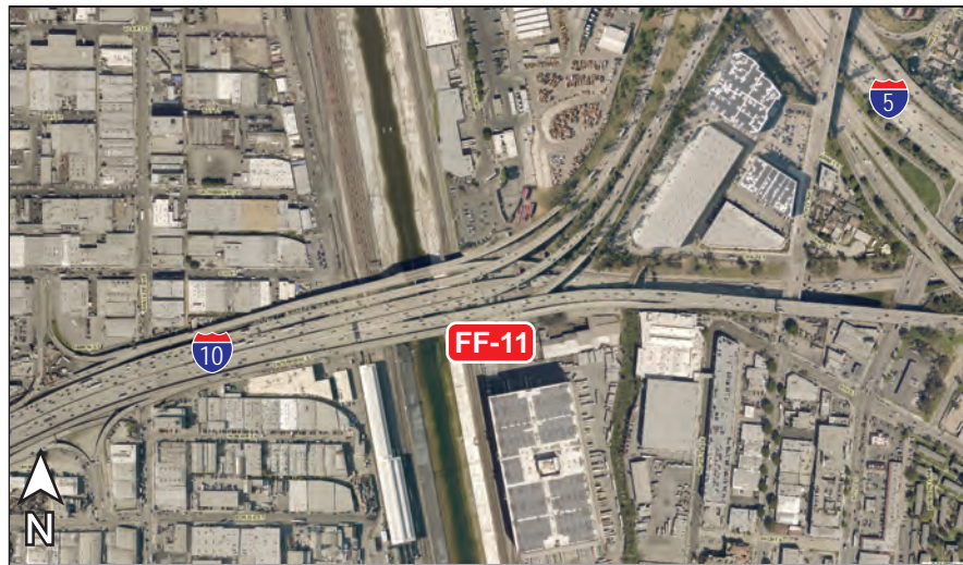
FF-11: I-10 East Lanes and Exit Ramp to SR-60 and I-5
