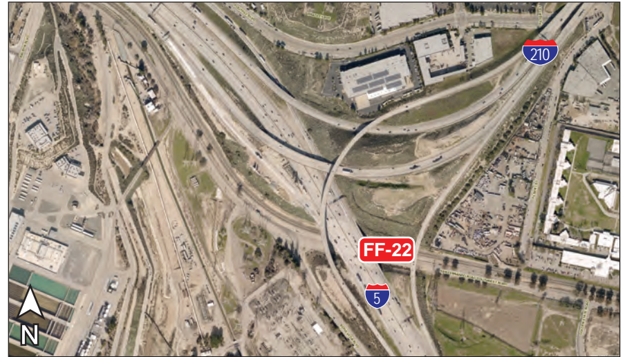
FF-22: I-5 North Lanes at San Fernando Road
