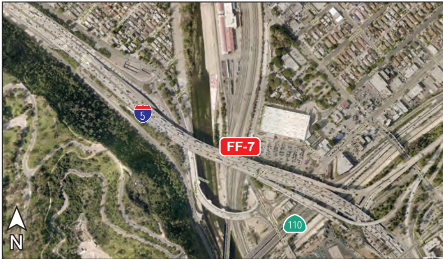
FF-7: I-5 North Lanes at San Fernando Road
