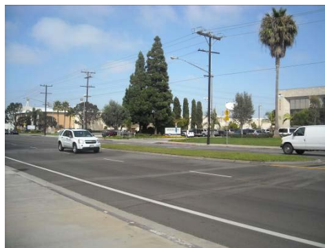
Figure 2-12. View of existing industrial uses along Redondo Beach Avenue
