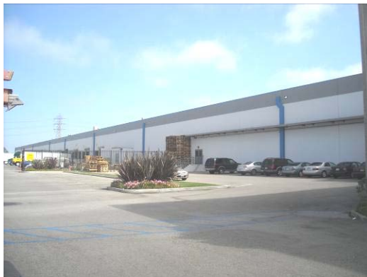
Figure 3-20. View of industrial warehouse on the site
