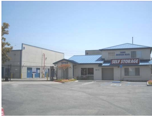
Figure 3-24. View of public storage facility on the site.
