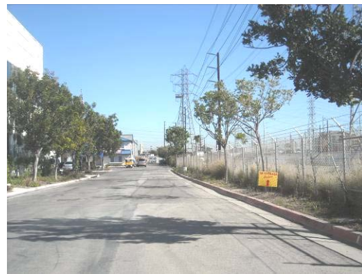
Figure 3-27. View of utility easement to the south of the public storage facility.
