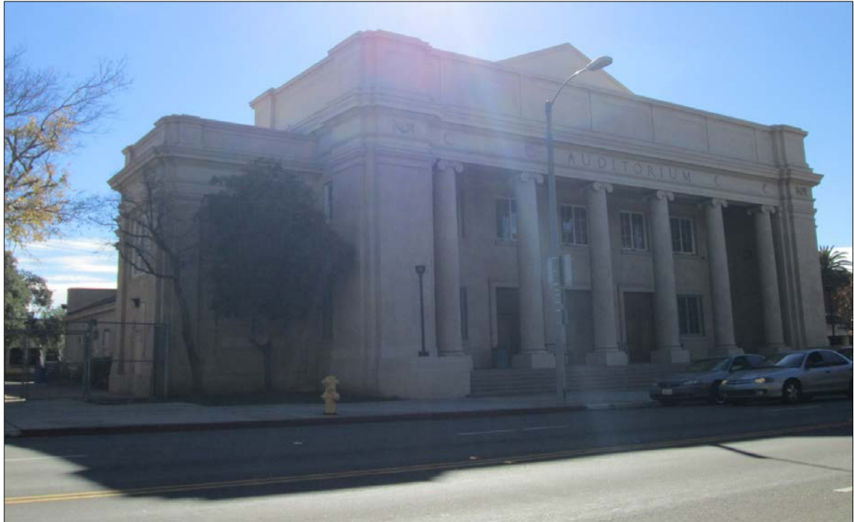
Figure 3-2: 130 N. Brand Boulevard, Auditorium, view looking southwest
