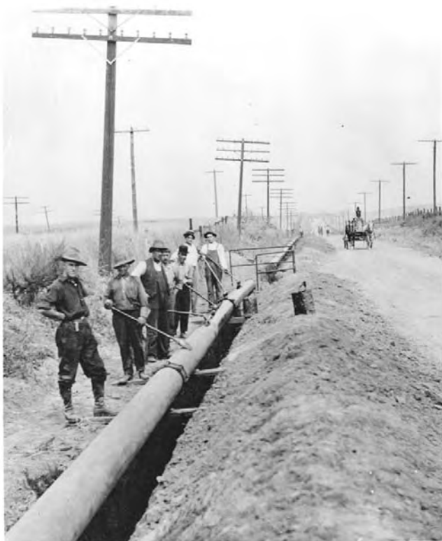
Gas line along San Fernando Road, 1910 CSUN Oviatt Library Digital Collection - San Fernanro Valley History Digital Library
