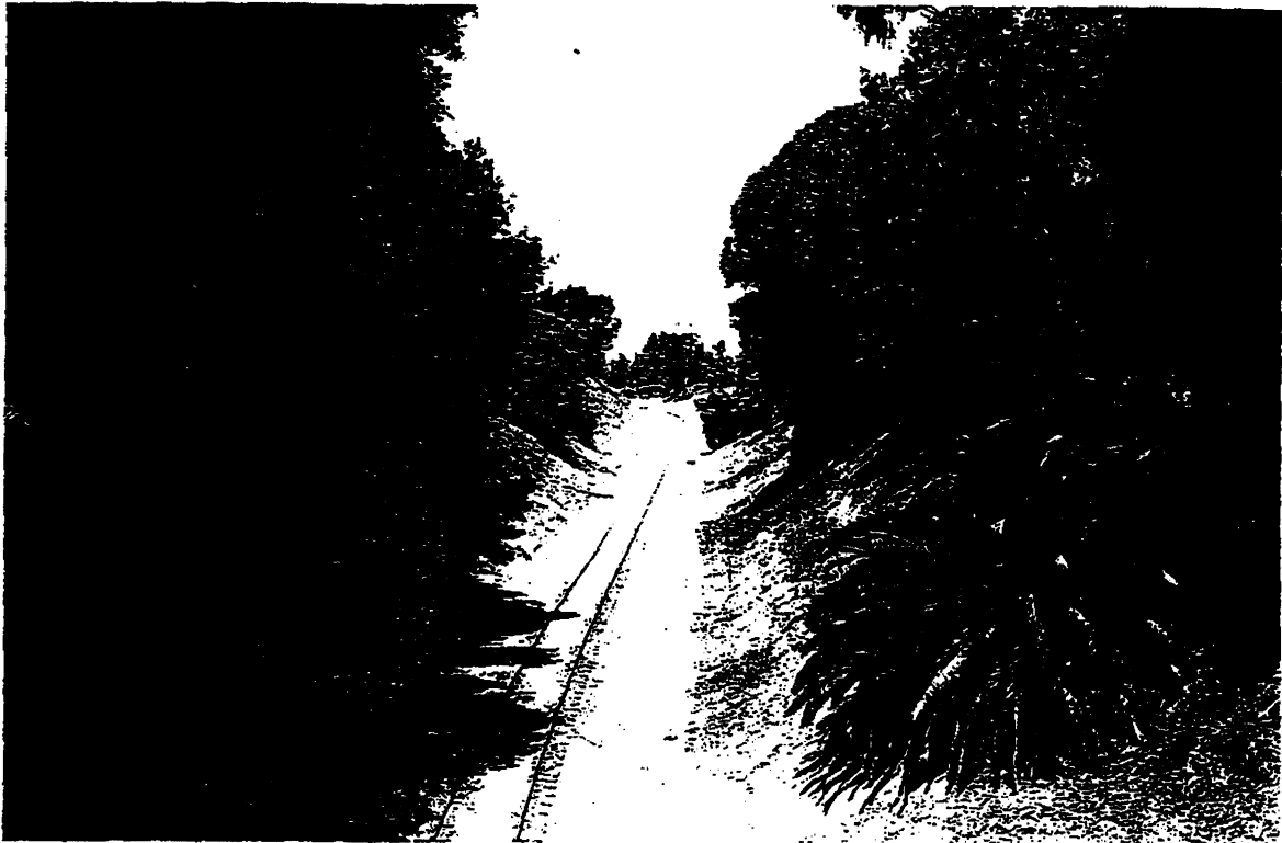
MOTOR AVE. WEST TO OVERLAND AVE. BELOW GRADE
