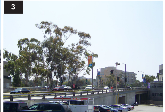
3 4th Street north of I-10 Looking Northwest
