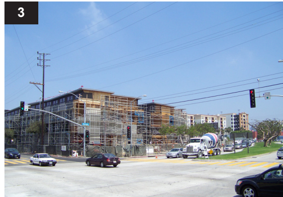
3 Olympic Boulevard at 20th Street Looking North
