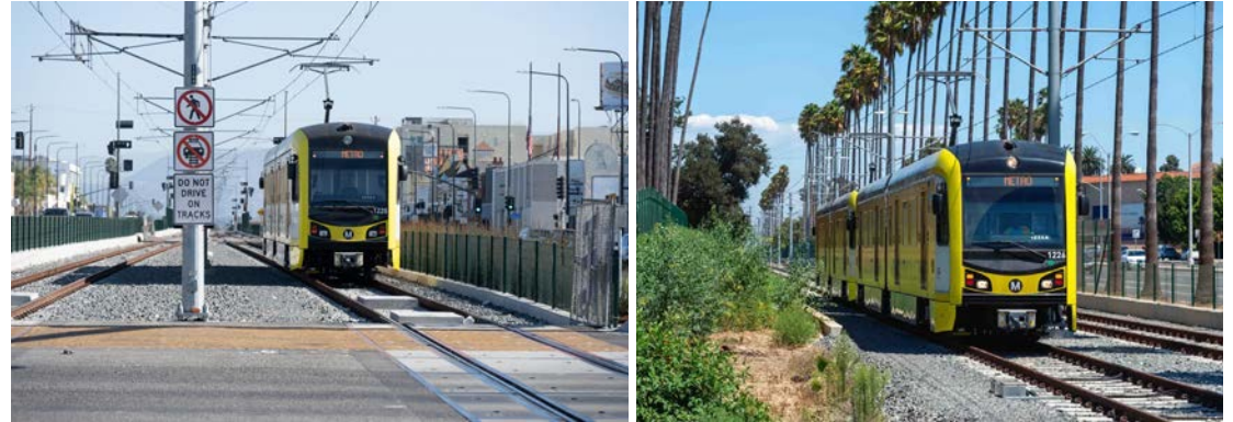
Elevated (Aerial) Guideways on Structural Columns and Retaining Walls
