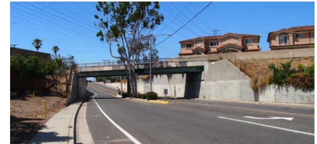
Existing Freight Bridge on Grant Ave, Looking West
