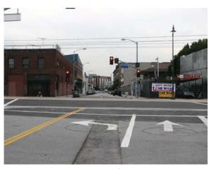
Photo 24 – The corner of 1<sup>st</sup> Street & Hewitt Street is a four-legged intersection. Pedestrian crossings are allowed across all intersection legs.
