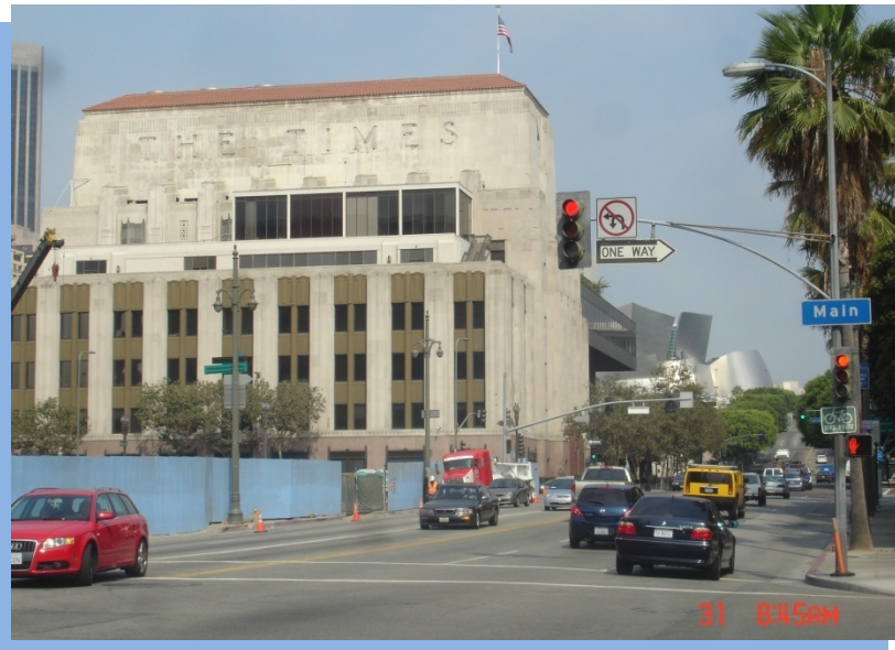
Figure 4.4-3. 1 st Street Corridor and the Los Angeles Times Building
