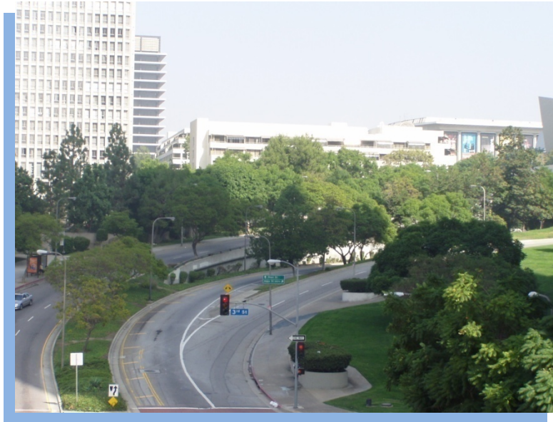
Figure 4.4-2. Open Space at West End of 2 nd and 3 rd Street Tunnels
