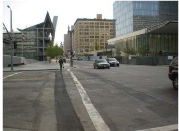
Photo 22 – 1 st Street and Main Street exhibit marked pedestrian crosswalks on all four legs to the intersection. The intersection is near City Hall.
