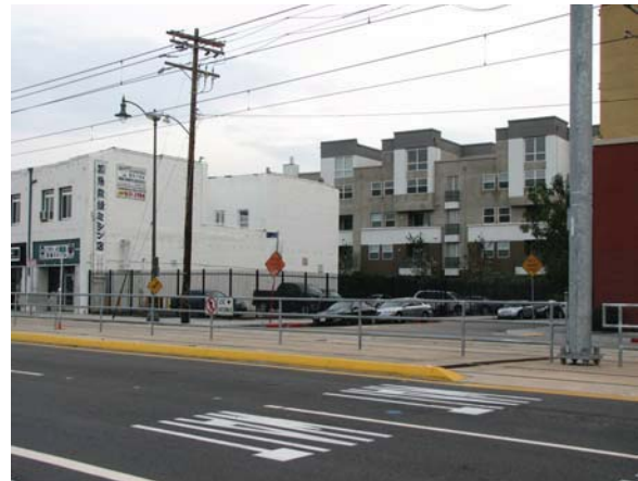
Photo 23 – 1 st Street and Rose Street is a “T” intersection. The Metro Gold Line traverses in an east-west direction (behind rail in photo).
