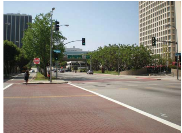
Photo 4 - The Flower Street and 3 rd Street intersection has excellent sight distance and is very open. The east leg begins the uphill grade to Bunker Hill.
