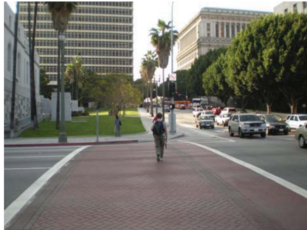
Photo 20 – The intersection of Temple Street and Main Street is located in the general vicinity of City Hall, and vehicle queuing was observed to back up into pedestrian crosswalks during the PM peak time – a potential safety concern.
