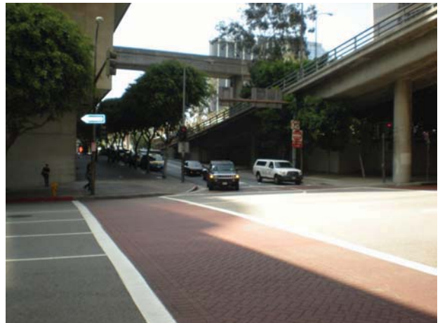
Photo 3 - The intersection of Flower Street and 4 th Street is essentially a "tee" intersection because the south leg serves a parking garage access. The overall intersection is dark with limited pedestrian sight distance due to bridge piers.
