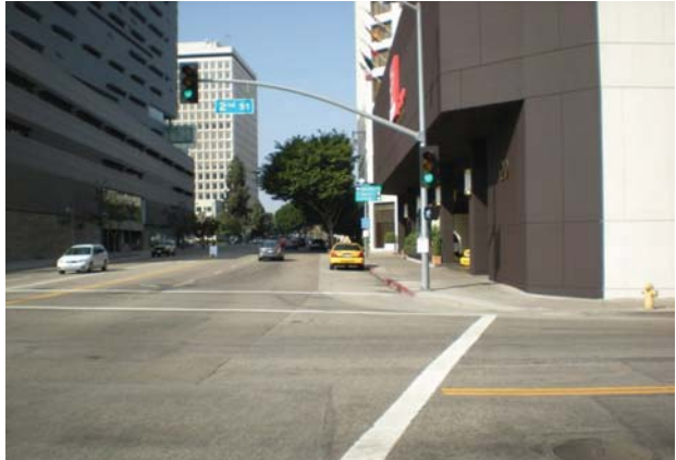
Photo 13 – 2 nd Street and Los Angeles Street is also adjacent to the Caltrans building. All legs of this intersection have marked crosswalks of inconsistent widths.
