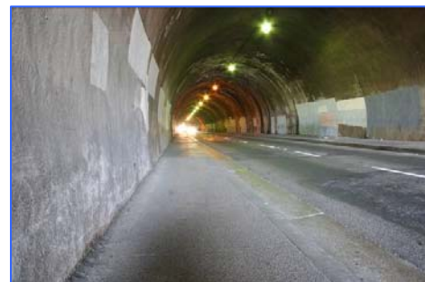
Figure 2-6 3 rd St. Tunnel
