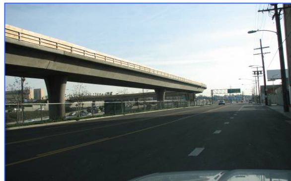
Figure 2-4 LRT Bridge over US-101
