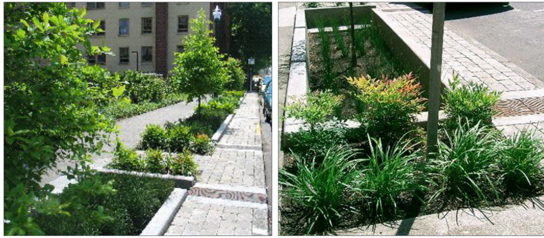
◀ Rain gardens collect water from impervious surfaces to support landscaped planters.
