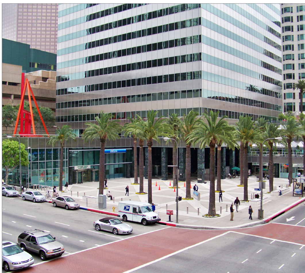
◀ Financial District – Existing Plaza
