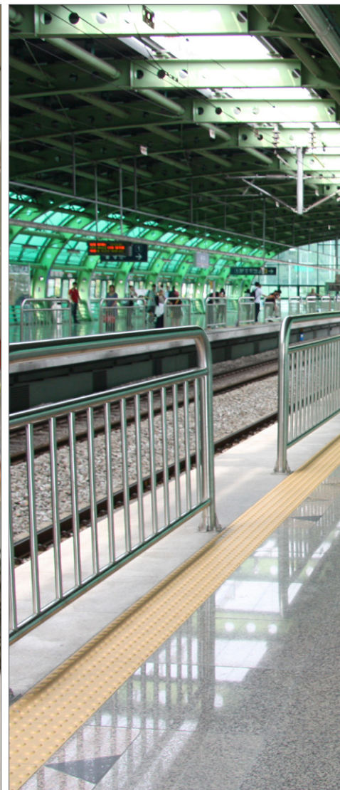
◀ Platforms must provide safe and clear circulation routes between trains and exits.
