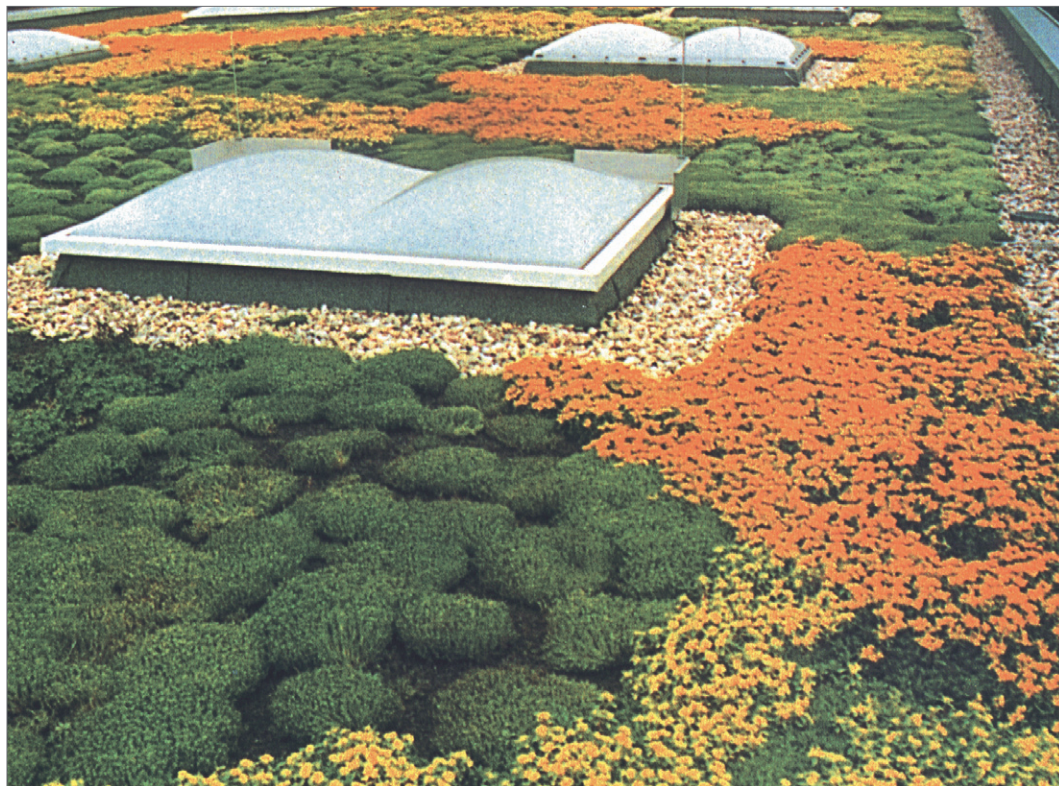
◀ Green roofs absorb energy from the sun and cool the building below.
