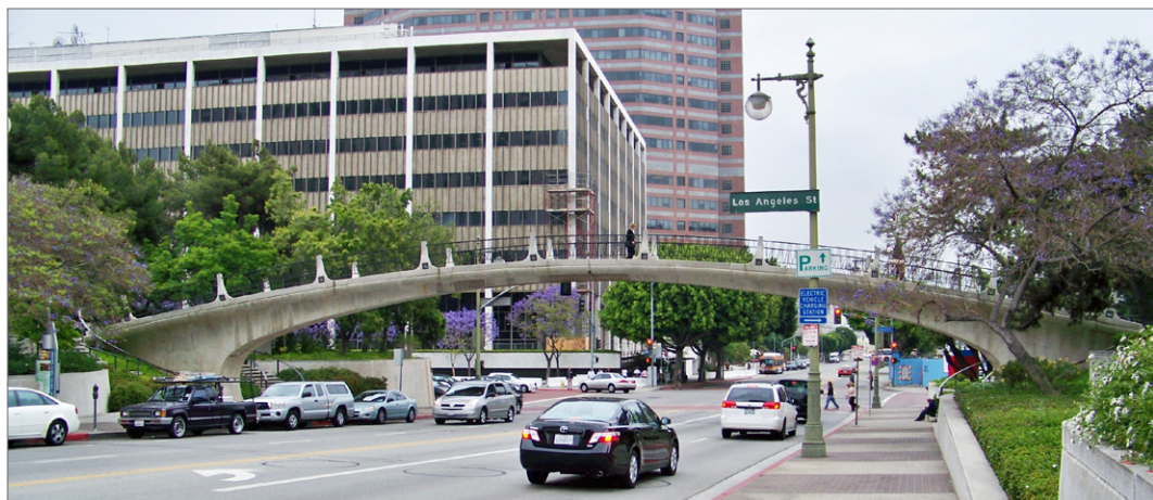
◀ Historic Core / Little Tokyo District – Existing Pedestrian Bridge
