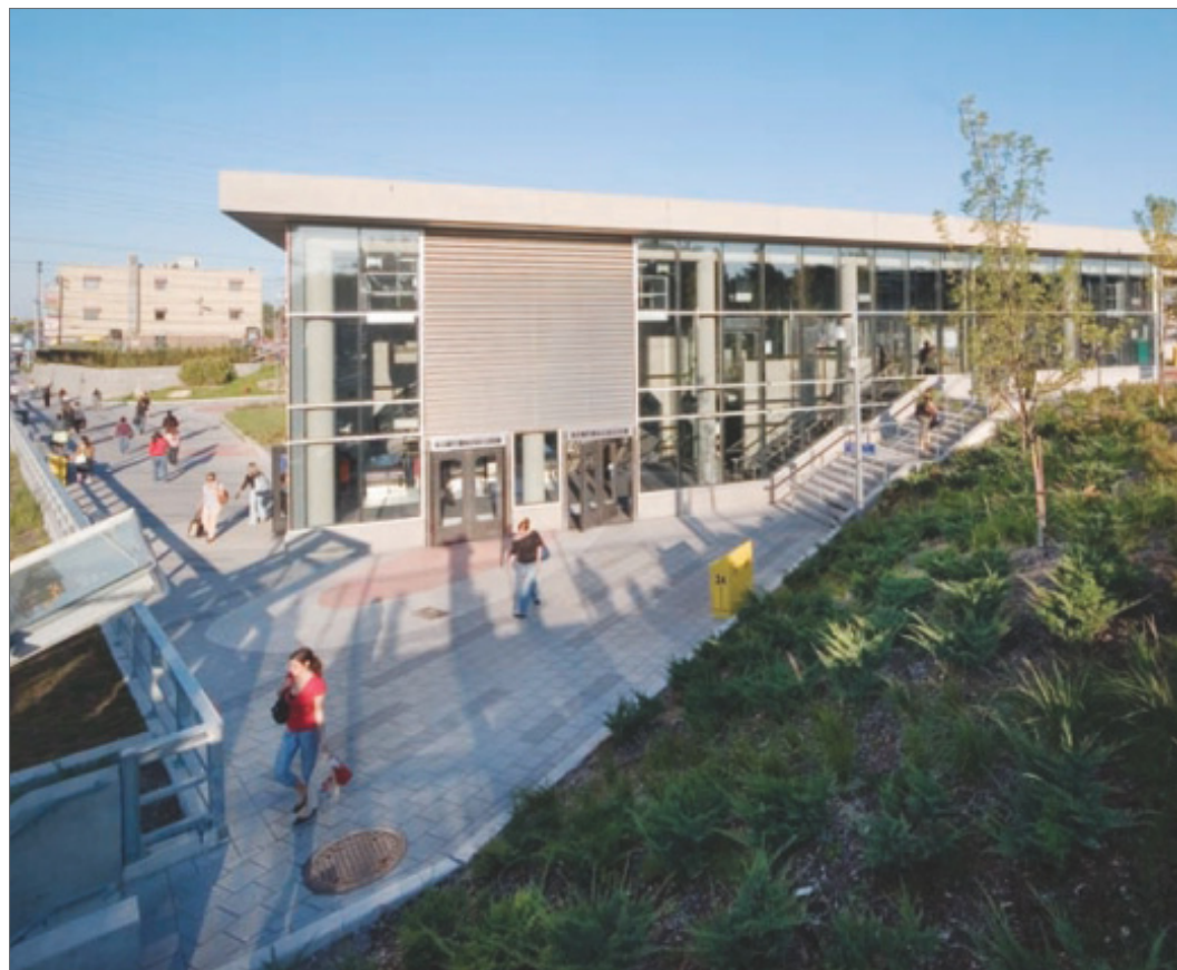
◀ Precedent - de la Concorde Transit Station, Laval QB
