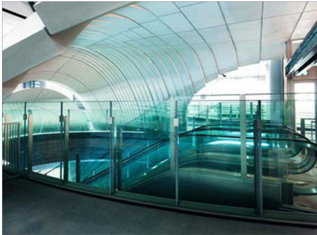
◀ Stations can be designed to provide natural ventilation with minimal equipment, like this station in Tokyo, Japan.
