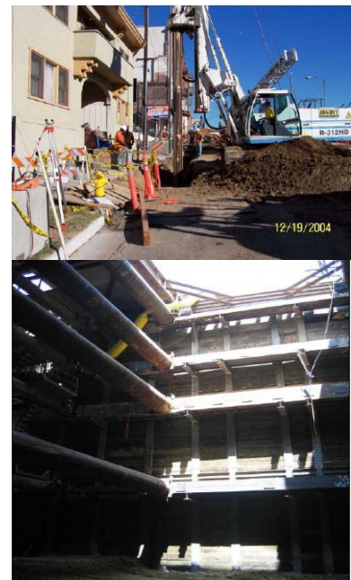
Figure 2-2. Typical Cut and Cover Construction Activities
