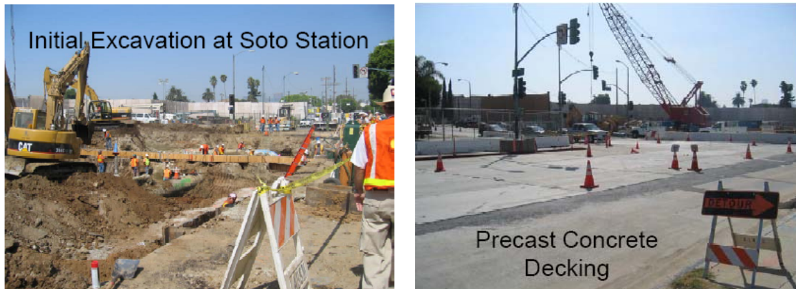
Figure 2-2. Typical Cut and Cover Construction Activities
