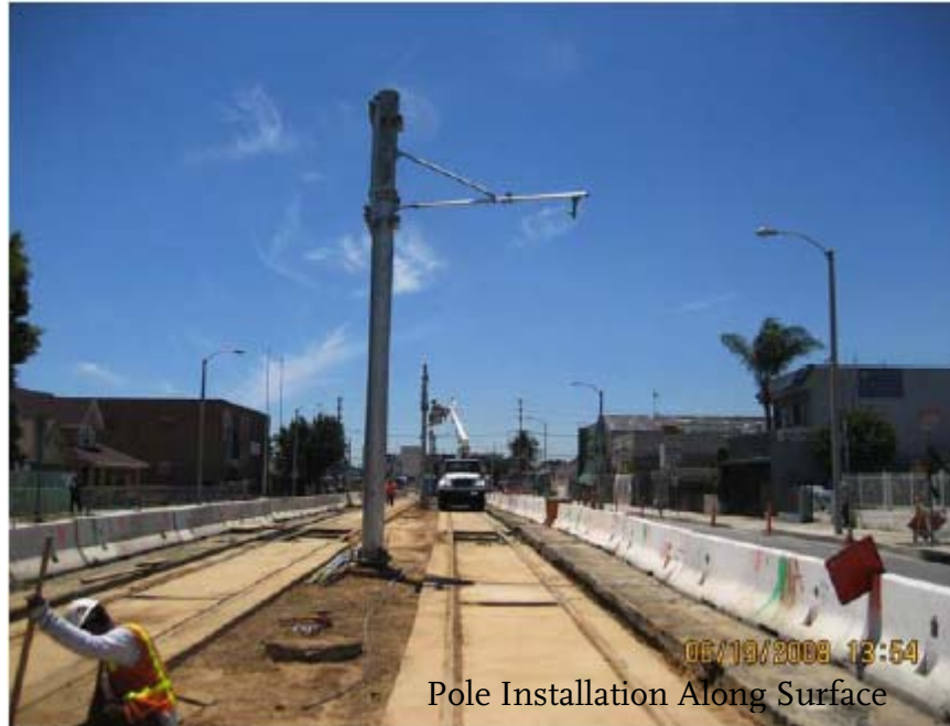
Figure 3-4. Typical Drilling and Installation of Pole
