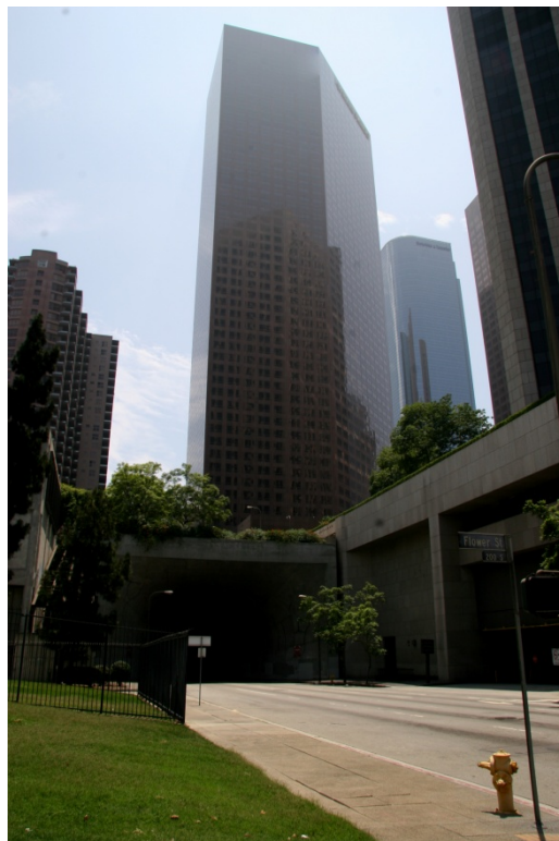
Figure 4-14. West End of 3 rd Street Tunnel
