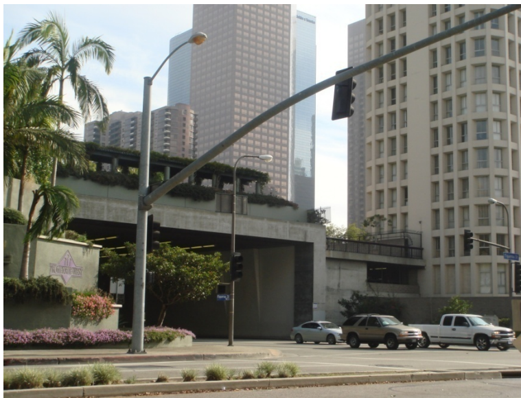
Figure 4-12. West End of 2 nd Street Tunnel
