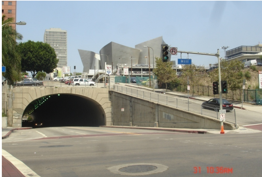
Figure 4-13. East End of 2 nd Street Tunnel
