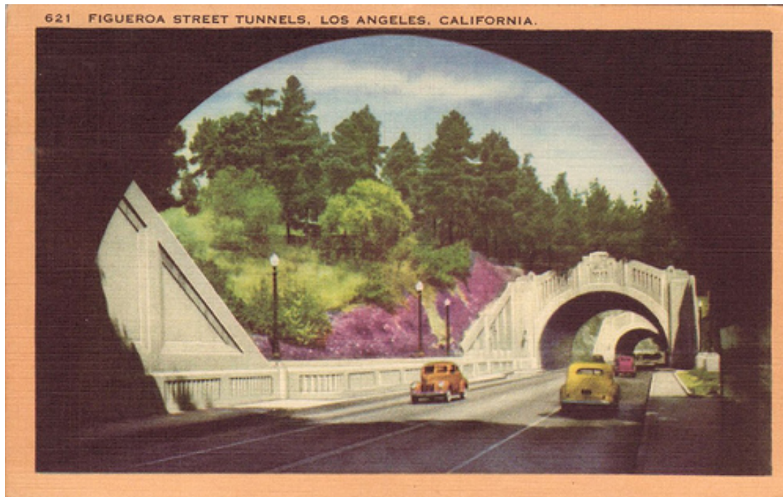
Figure 4-2. Figueroa Street Tunnels, view north, circa 1940s.
