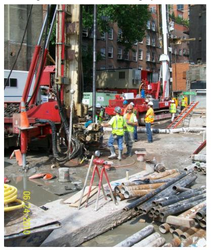
Figure 4-8: Surface Jet Grouting Operation
