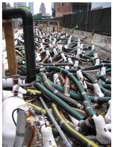
Figure 4-13: Freeze Pipe Array
