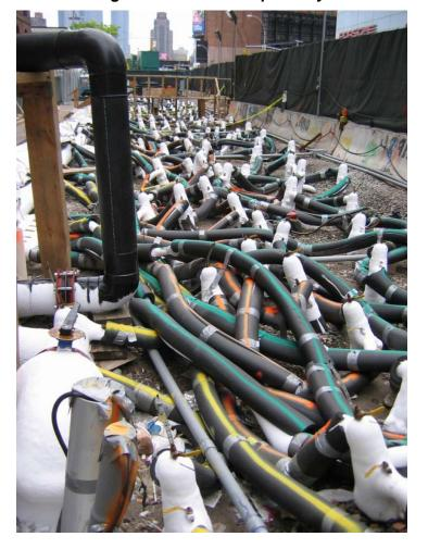
Figure 4-13: Freeze Pipe Array
