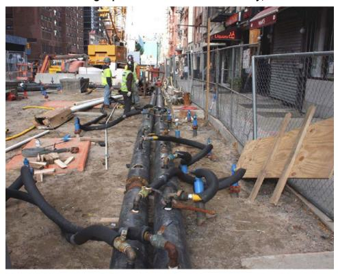
Figure 4-12: Ground Freezing Operation
