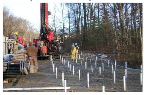
Figure 4-4: Permeation Grouting from Surface
