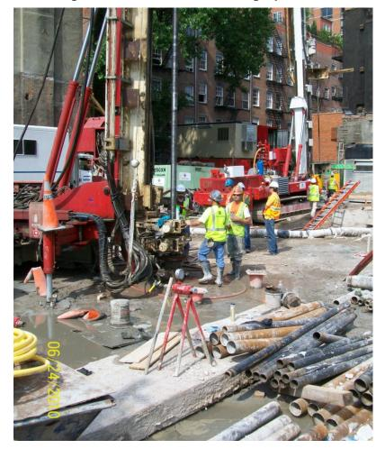
Figure 4-8: Surface Jet Grouting Operation
